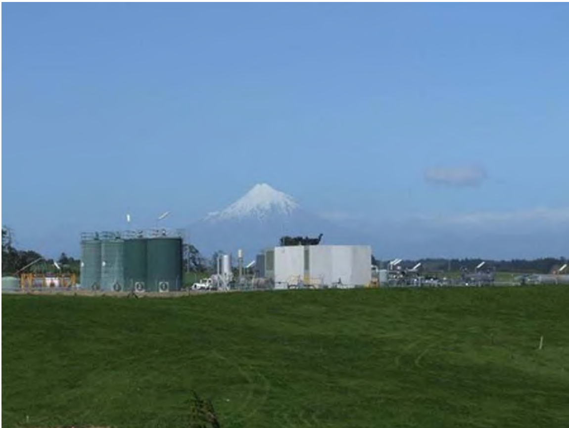
Photo 1 Turangi Production Station
