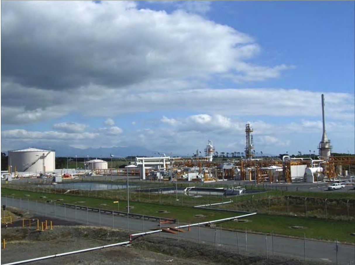
Photo 1 Pohokura Production Station
