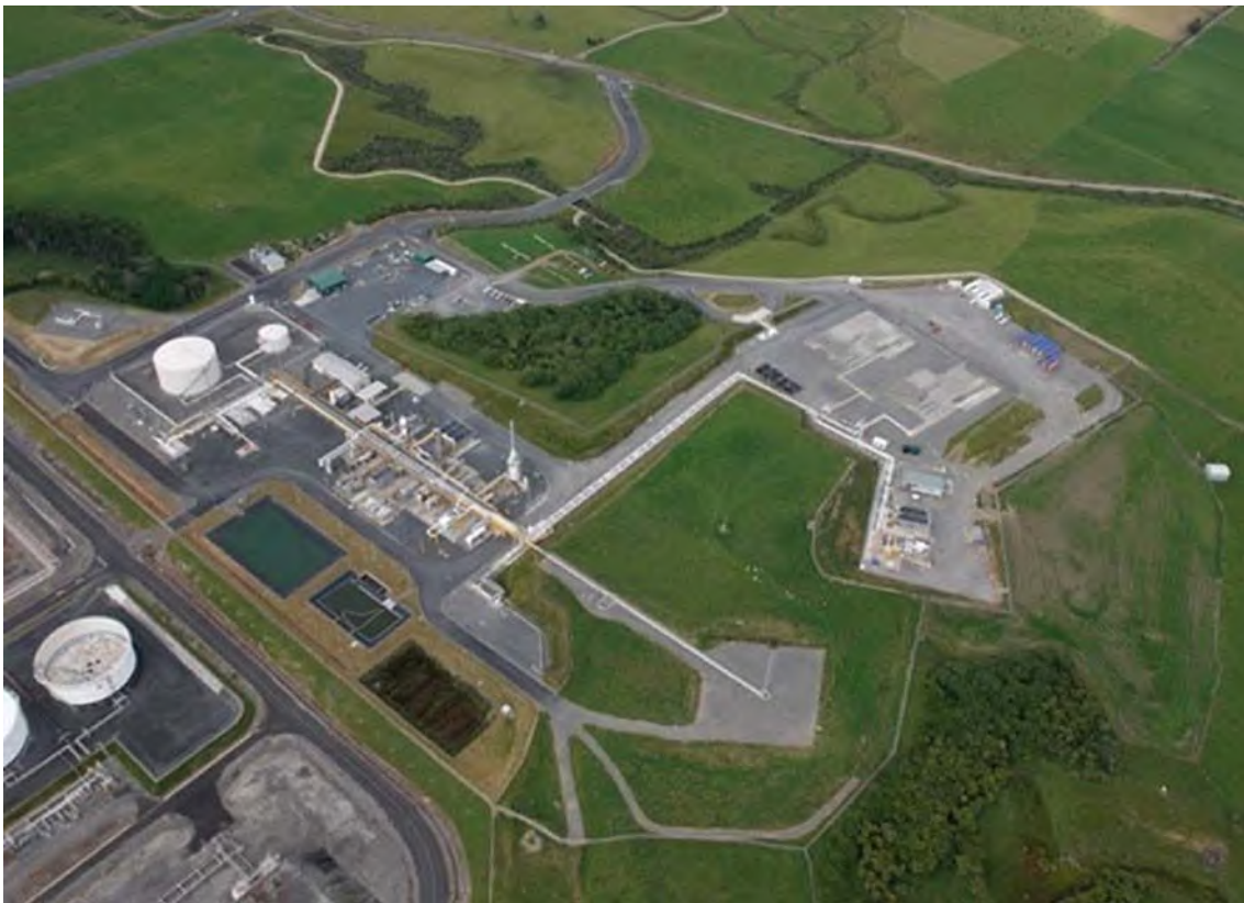
Photo 2 Aerial view of Pohokura Production Station.
