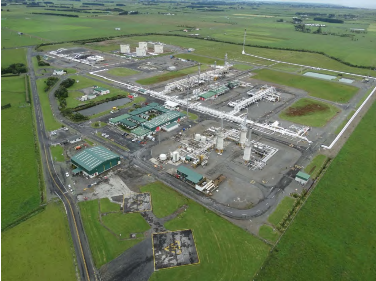
Photo 1 Maui Production Station
