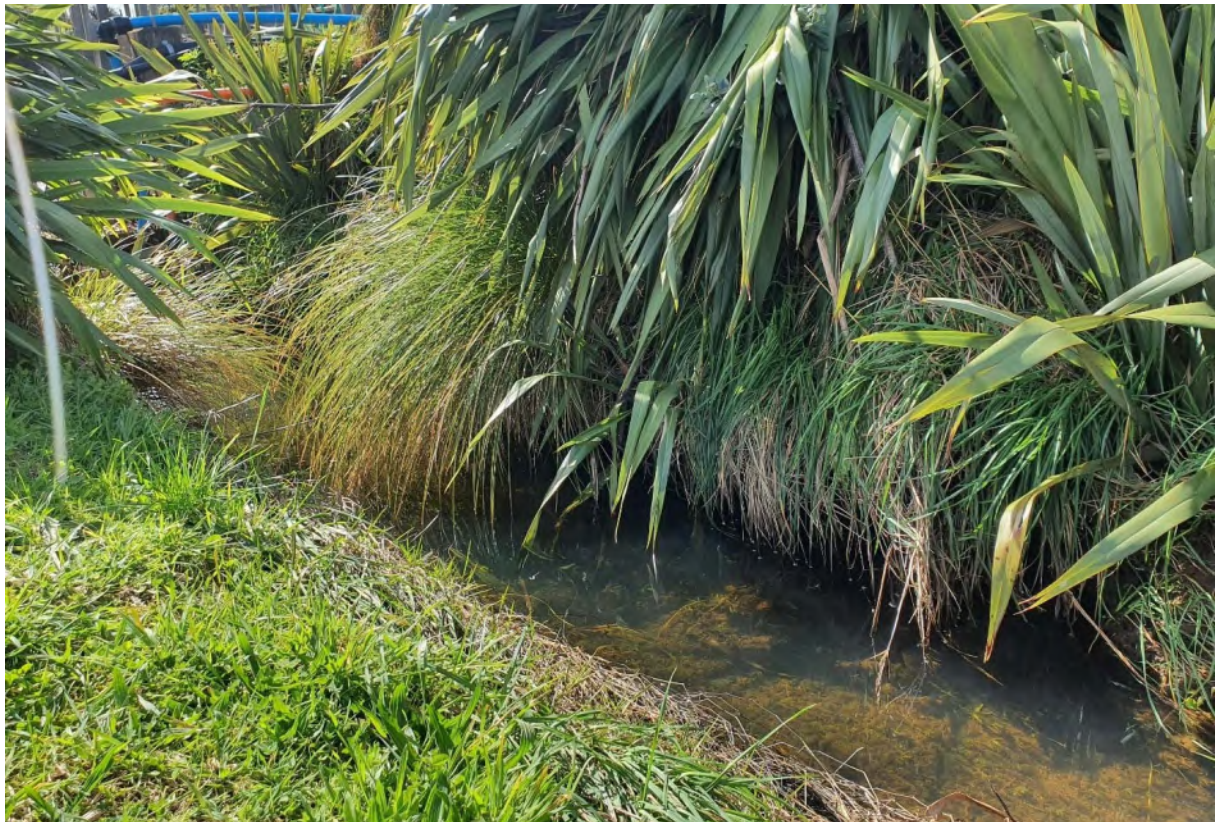
Photo 2 Combined discharge in the drain/tributary prior to entry into the Ngapirau Stream
