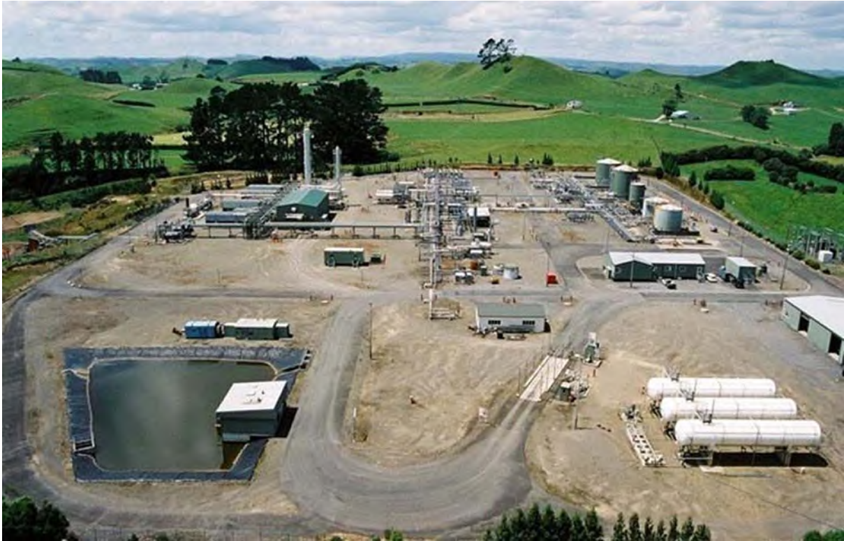
Photo 1 Waihapa Production Station
