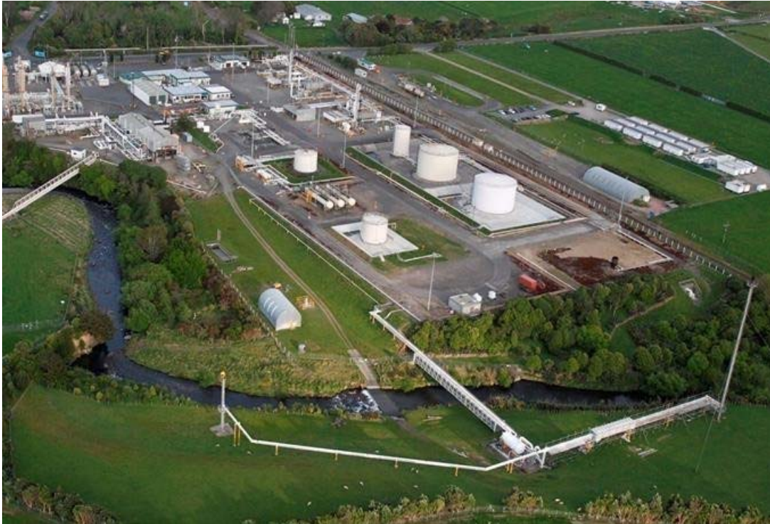
Photo 1 Kapuni Production Station
