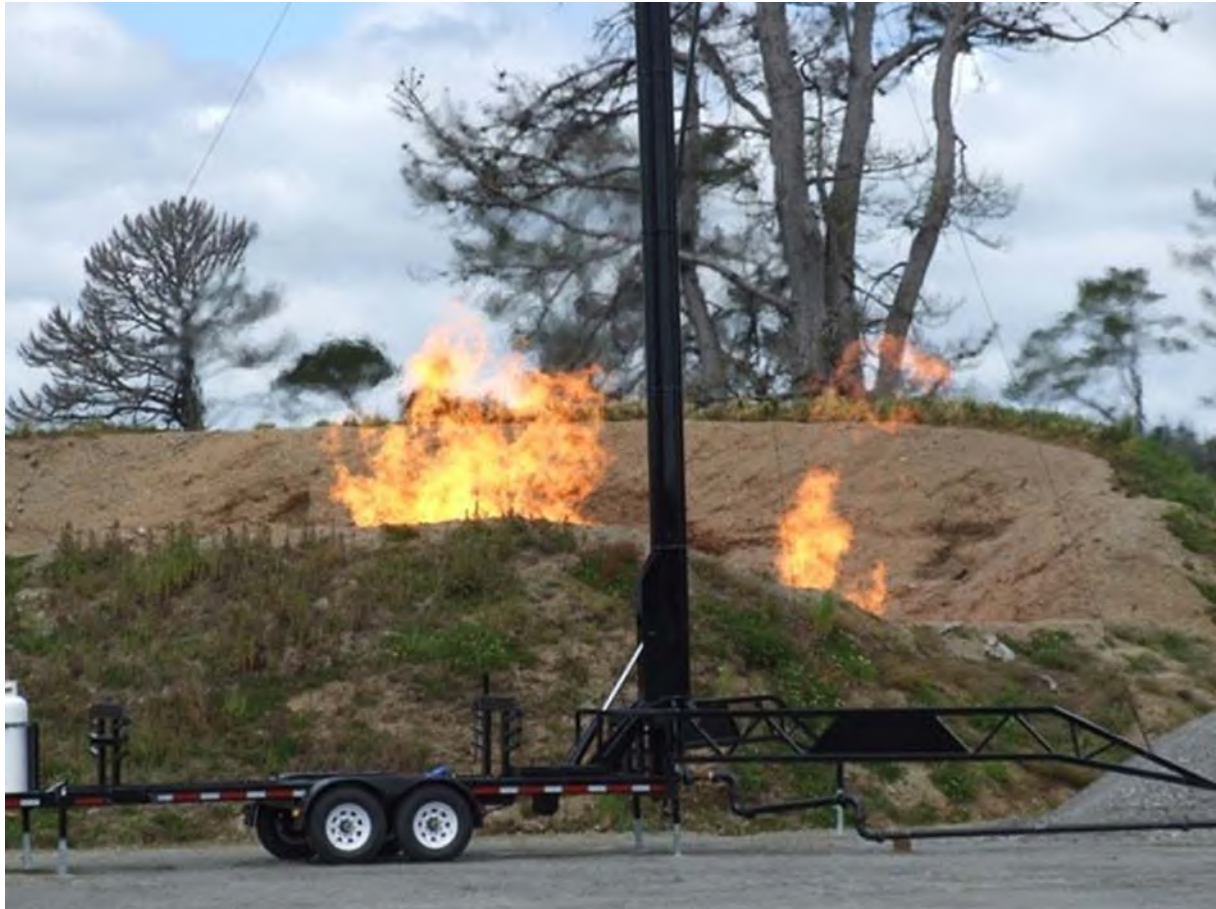
Photo 2 Clean burning flare at the Sidewinder Production Station
