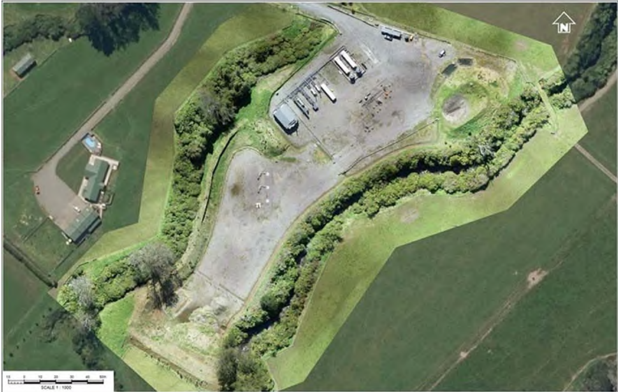
Photo 1 Sidewinder Production Station and wellsite (2019)
