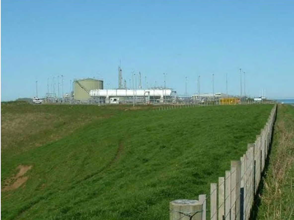
Photo 1 Rimu Production Station
