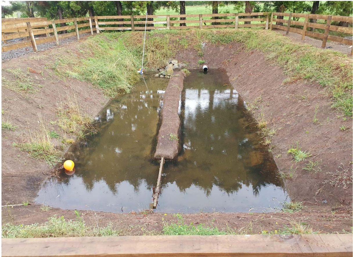
Photo 4 An additional unlined settling pond has been added in series with the existing two lined pits to further settle out suspended sediment prior to discharge
