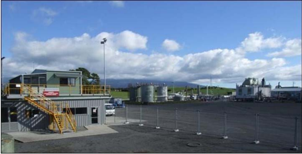
Photo 1 Kaimiro Production Station
