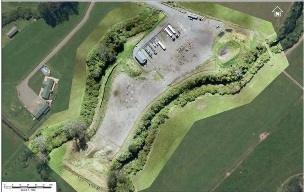
Photo 1 Sidewinder Production Station and wellsite (2019)
