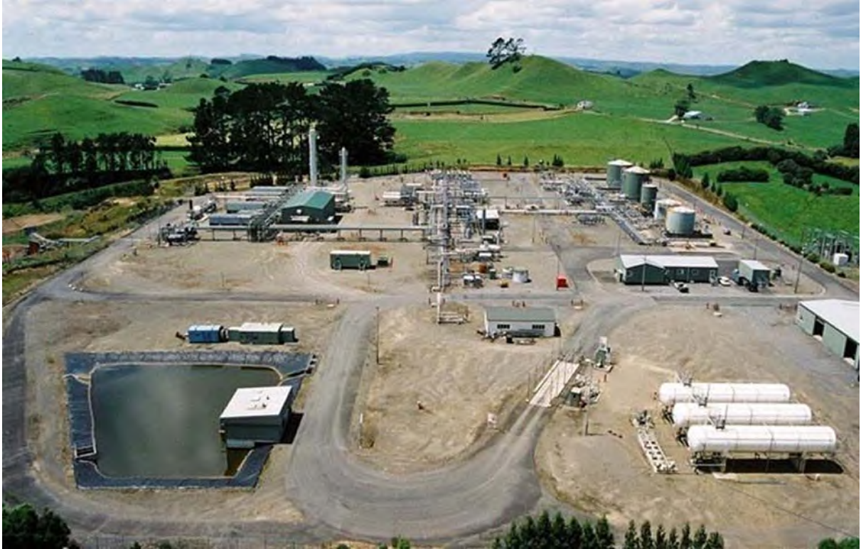
Photo 1 Waihapa Production Station
