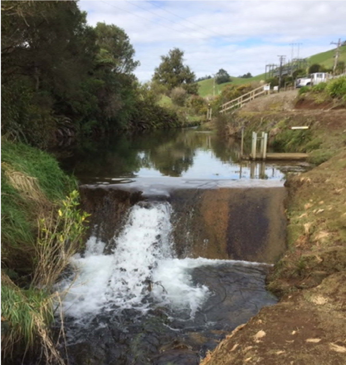
Photo 2 MMPS water supply weir in the Mangahewa Stream, the stepped fish pass is in the centre
