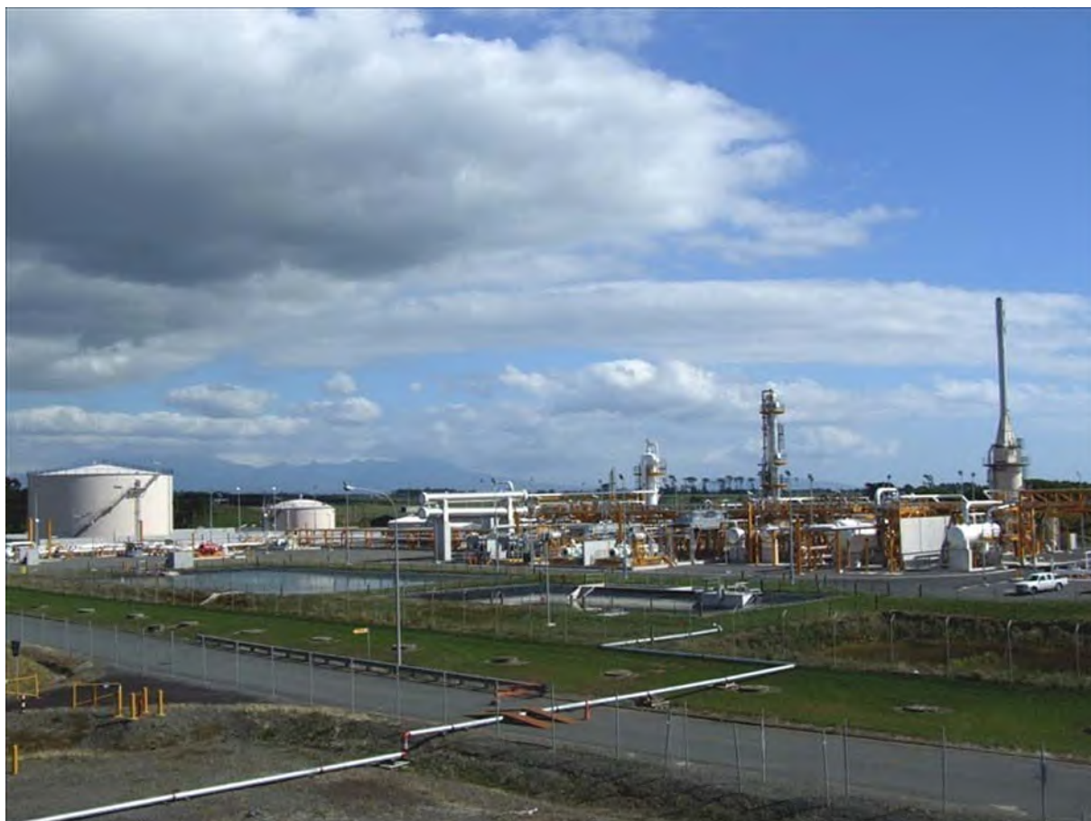
Photo 1 Pohokura Production Station
