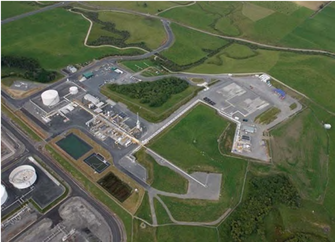
Photo 2 Aerial view of Pohokura Production Station
