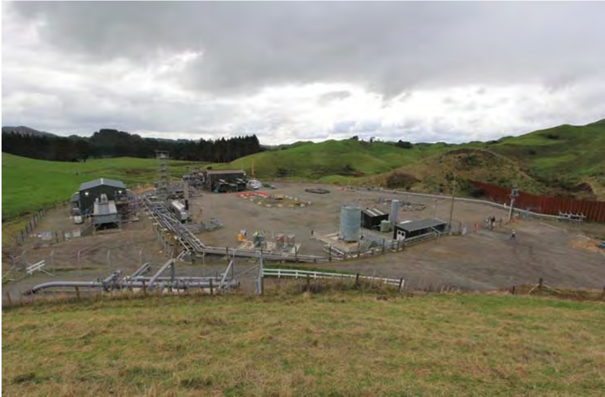
Photo 1 Ahuroa-B site layout facing North West, May 2014
