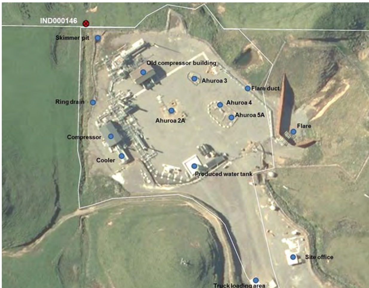
Photo 2 Ahuroa-B wellsite and gas storage facilities
