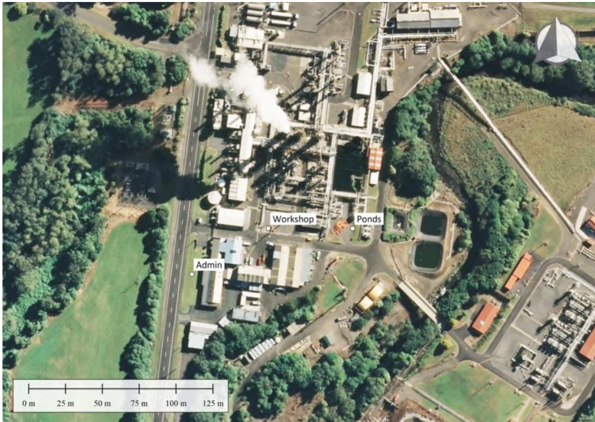
Figure 6.7: Metal deposition monitoring locations.
