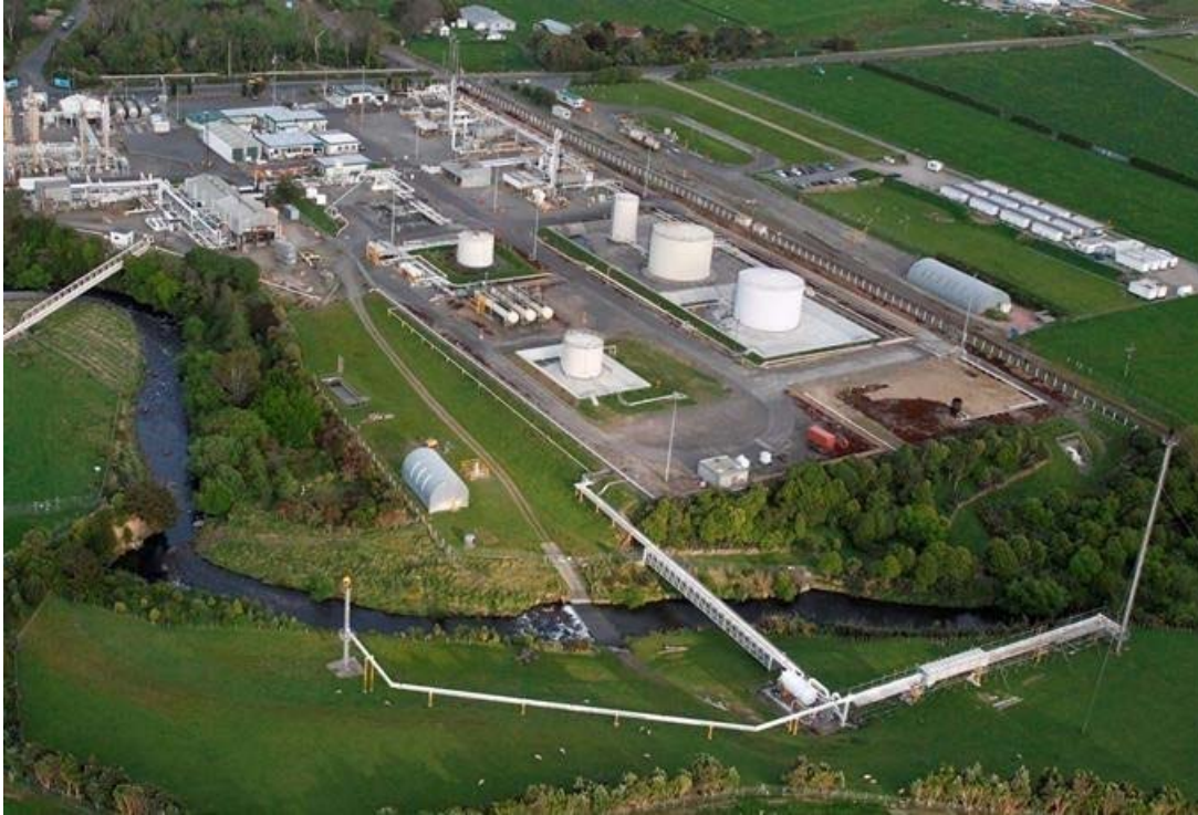
Photo 1 Kapuni Production Station
