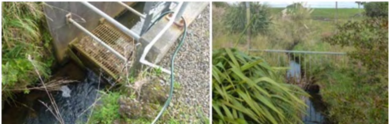
Photo 2 Discharge to the Ngapirau Stream
