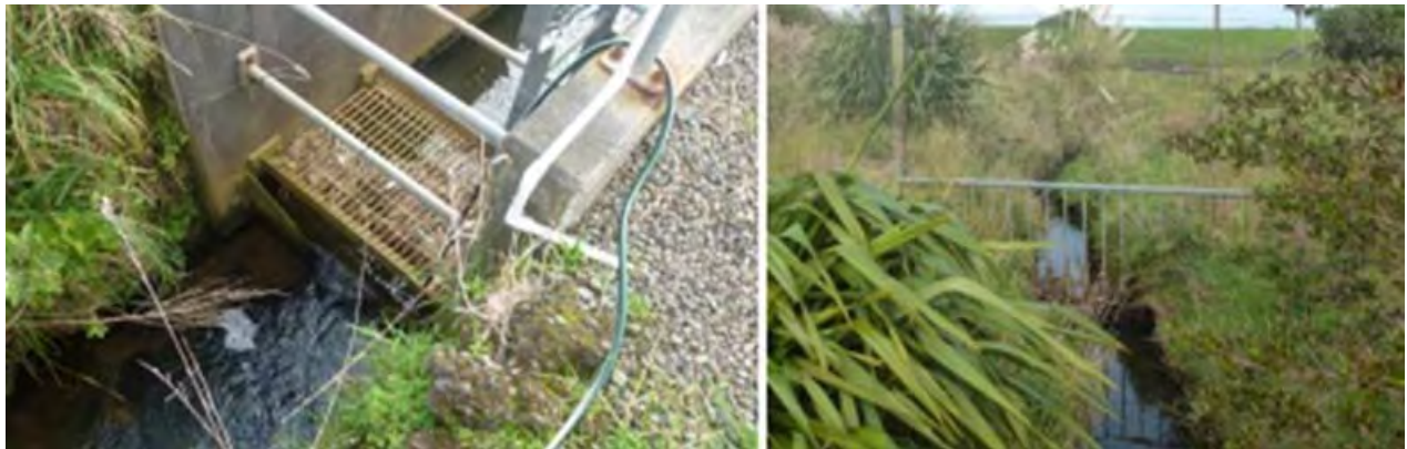
Photo 2 Discharge to the Ngapirau Stream
