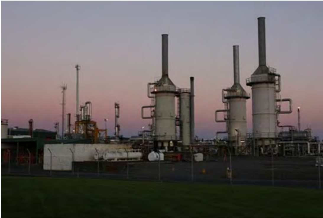
Photo 3 Emission sources at the Maui Production Station
