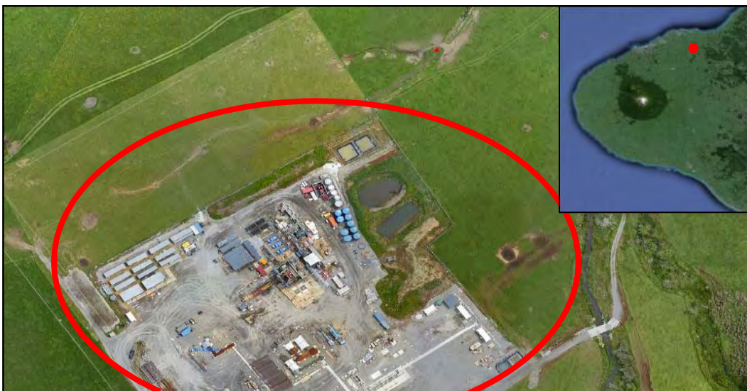
Figure 1 Aerial view depicting the locality of the Mangahewa-D wellsite, with approximate regional location (inset)
