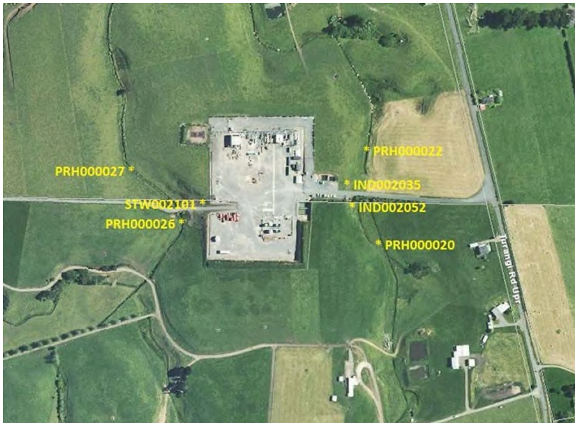
Figure 1 Turangi Production Station and associated sampling sites
