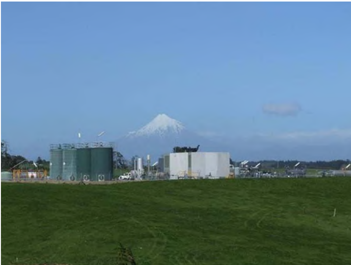
Photo 1 Turangi Production Station
