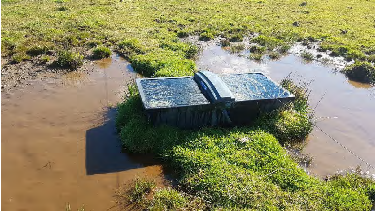
Photo 2 Overflowing water trough and surrounding ponding at Stratford landfill
