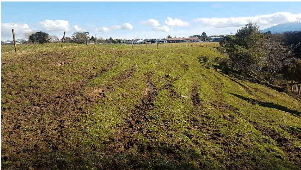
Photo 4 Example of stock damage to the batter at Stratford landfill
