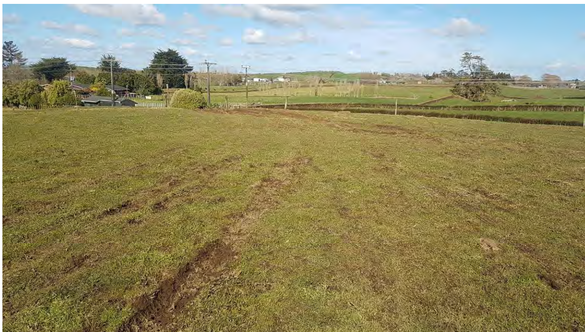
Photo 5 Example of vehicle and stock damage to the cap at Stratford landfill
