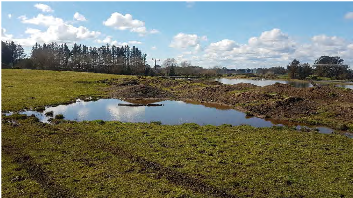
Photo 1 Area of ponding on the cap at Stratford landfill
