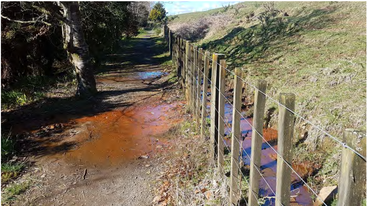
Photo 3 Stormwater/leachate/groundwater overflow from Stratford landfill across public walkway
