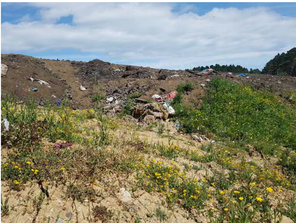
Photo 12 Insufficient cover, 20 December 2017
