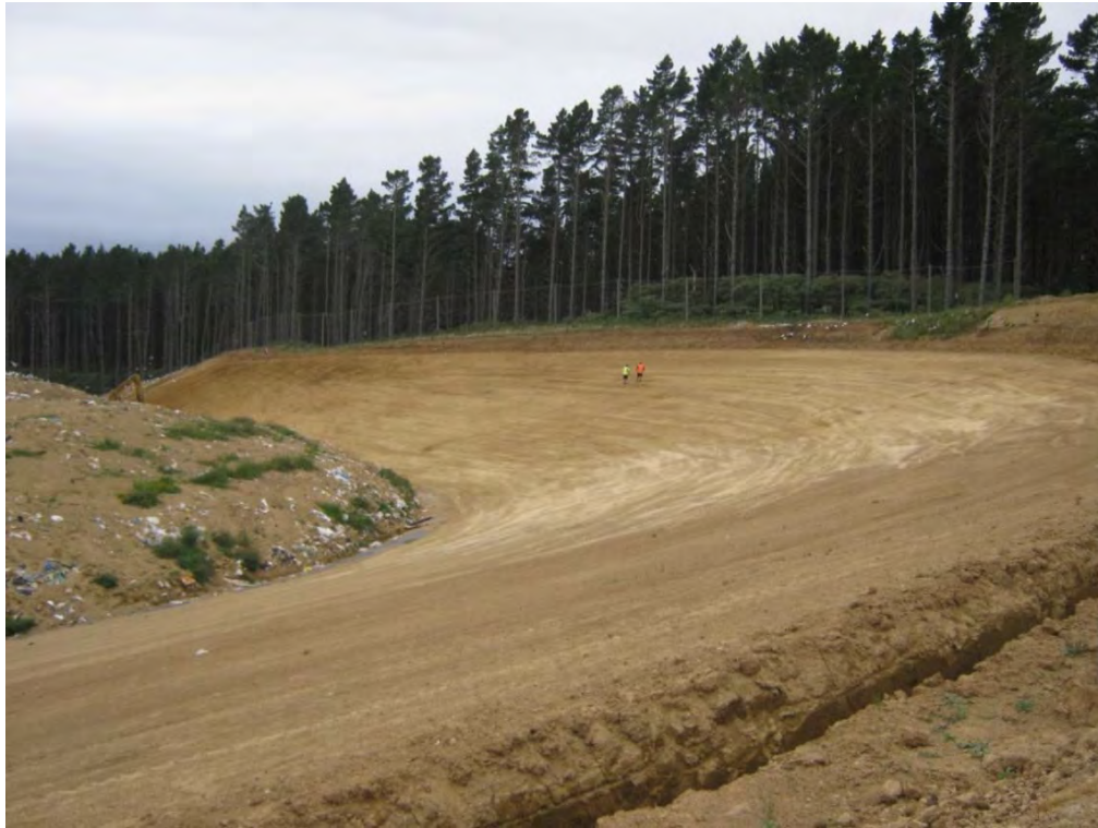
Photo 1 Stage 3 extension works, February 2011
