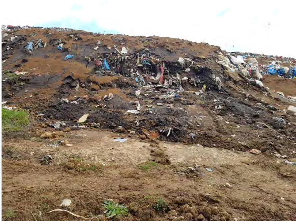
Photo 9 Cover slumping, 4 October 2017
