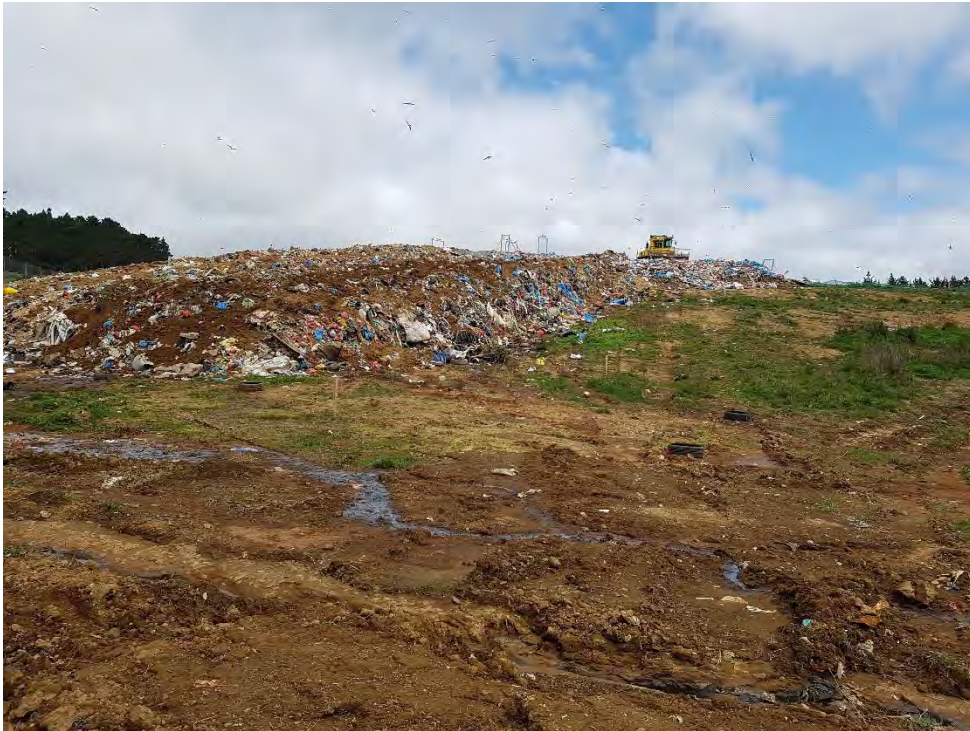
Photo 11 Insufficient cover, 4 October 2017
