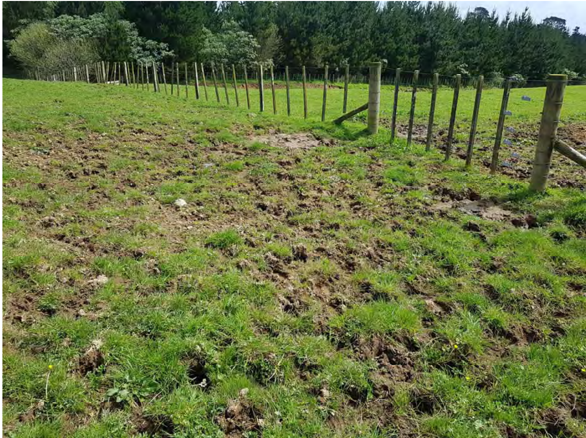
Photo 4 Stage 2 cap condition at inspection on 4 October 2018
