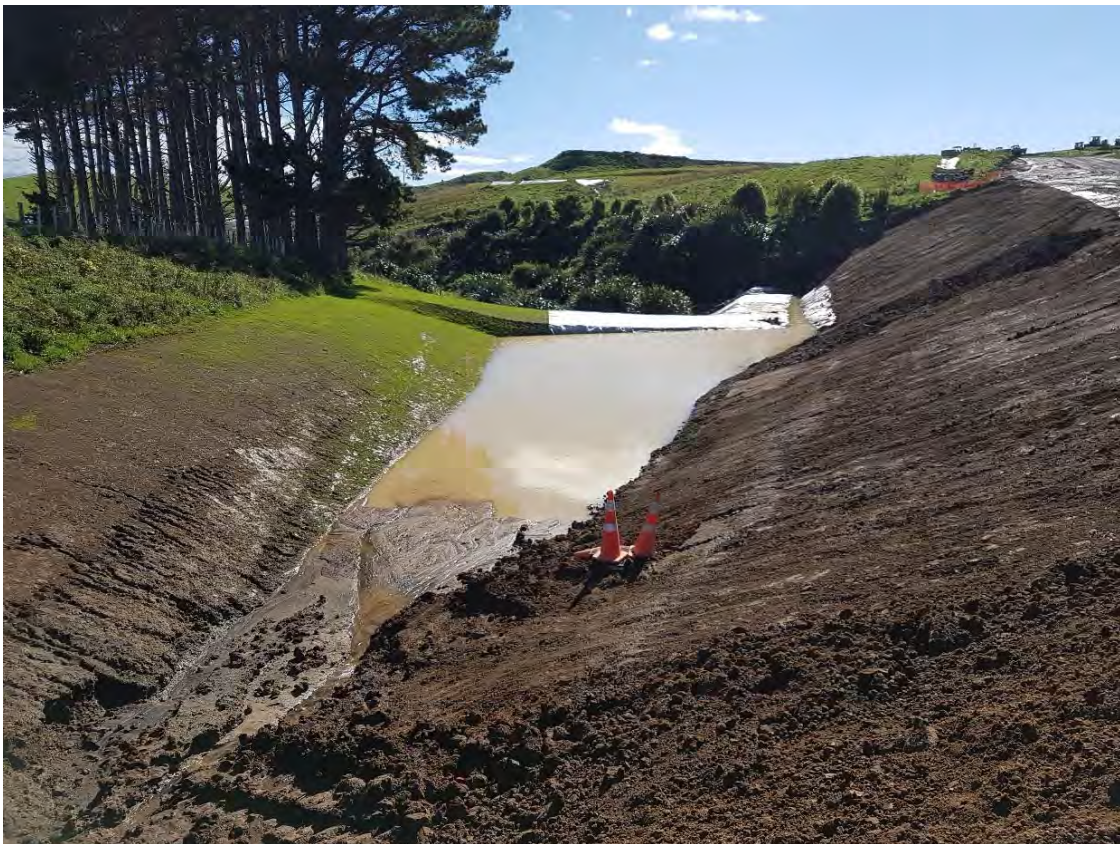
Photo 9 Silt controls above southern ephemeral tributary, May 2018
