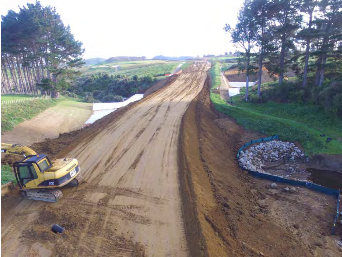
Photo 6 Southern access track, culvert and silt controls, April 2018
