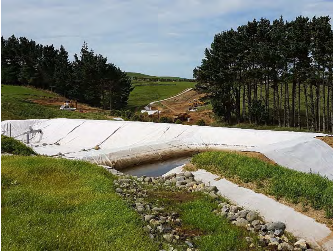
Photo 8 Silt controls below the stockpile area in the north west corner of the site, March 2018
