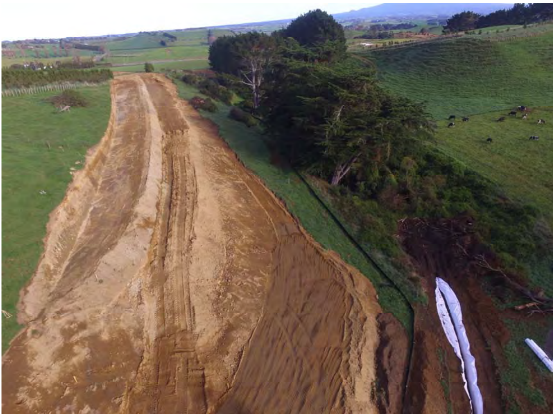
Photo 7 Access track and silt controls, April 2018
