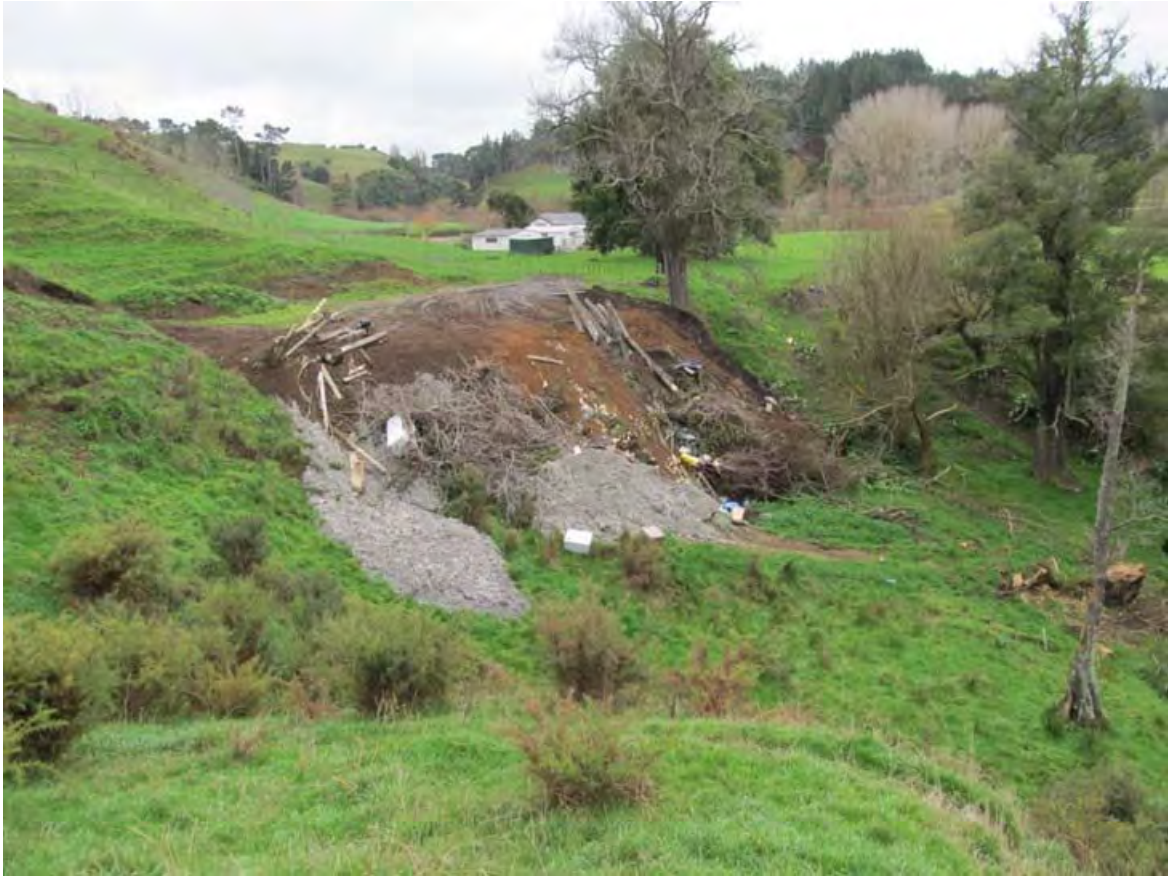
Photo 1 Photograph showing the refuse dump prior to capping
