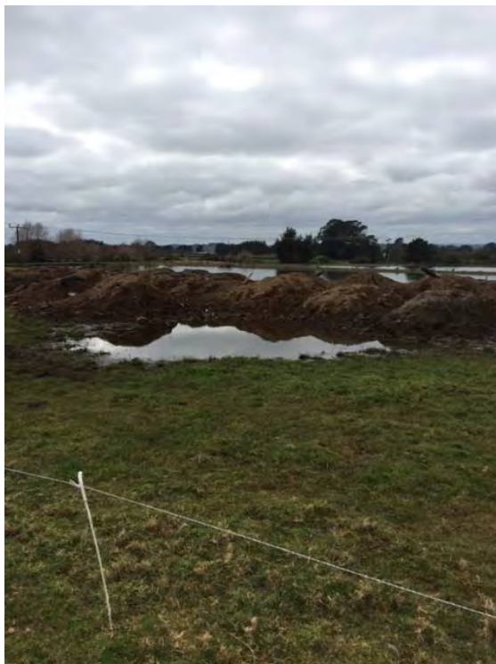
Photo 1 Recontouring material and ponding on cap, 01 Sept 2016
