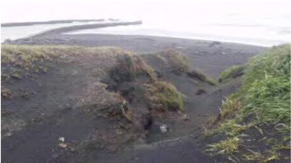
Photo 3 Stormwater erosion found at inspection on 22 October 2015
