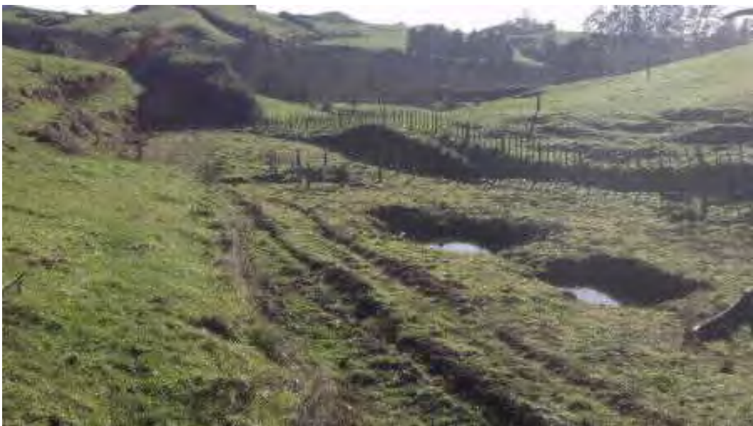
Photo 2 Silt ponds and vegetative cover establishing at lower end of stage 2 basin
