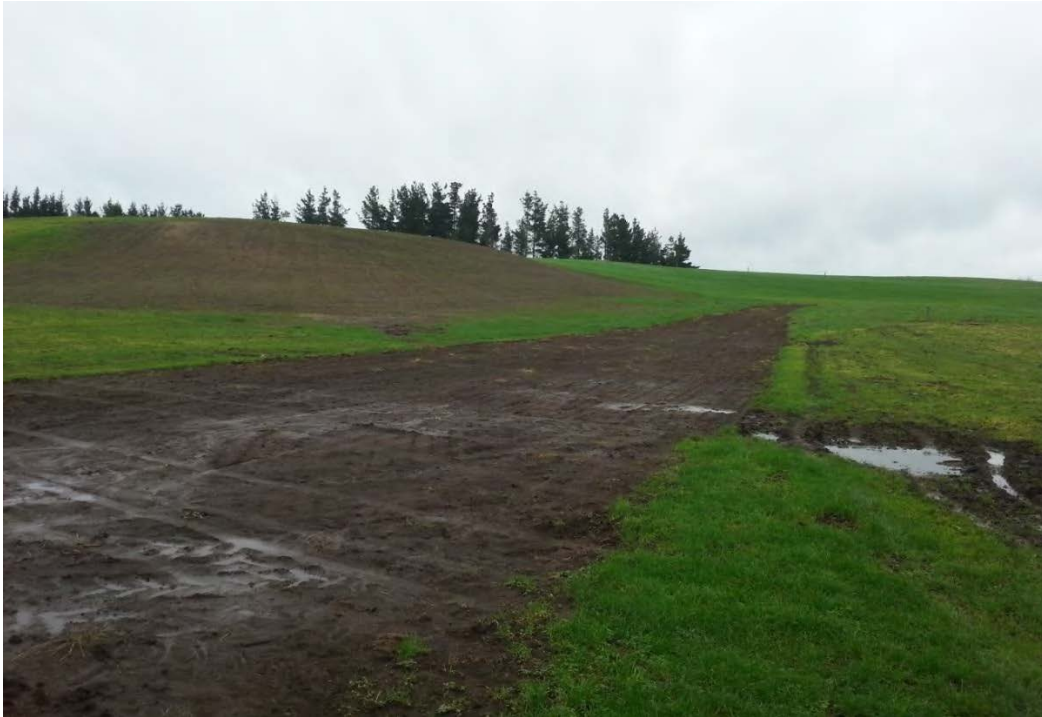
Photo 5 Fresh soil in scraped out area and re-contoured burial area (at rear)
