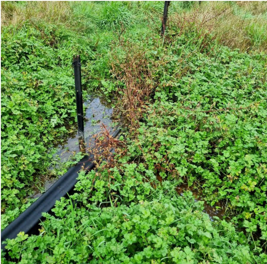
Photo 3 One of the silt fences needing to be reinstated
