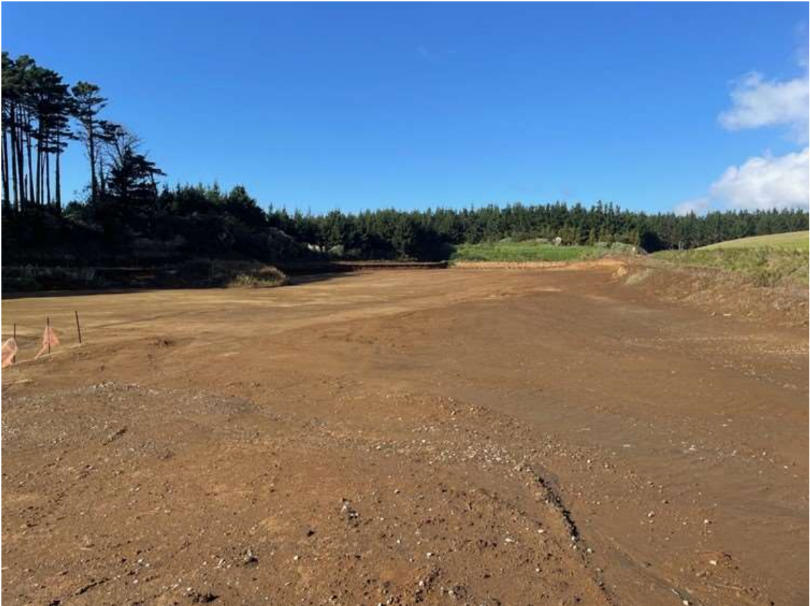
Photo 9 Borrow area stabilised for the winter by compaction, May 2024
