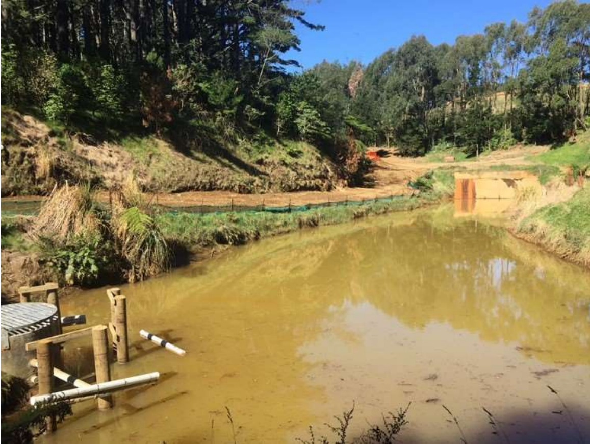
Photo 6 Floating decant system in the large silt pond, April 2024
