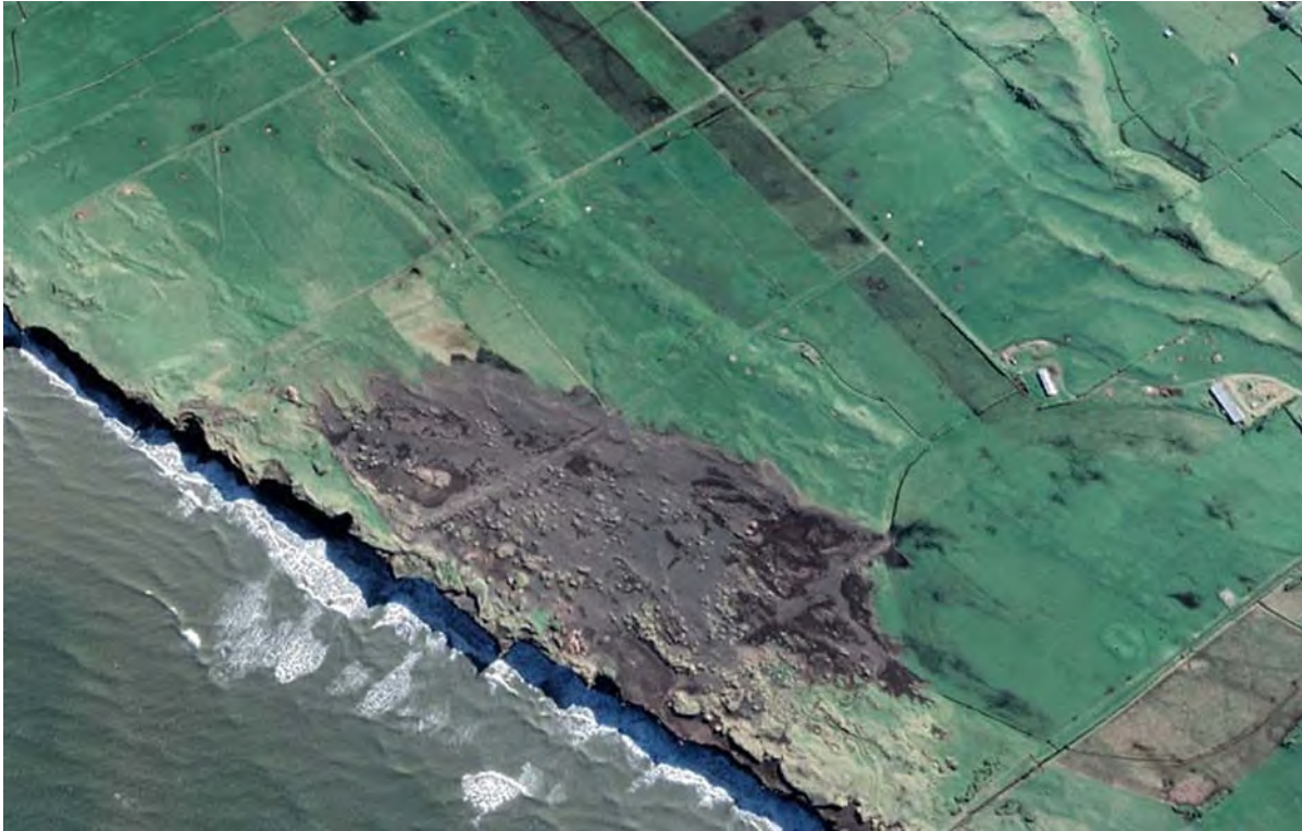
Figure 6 Aerial image showing the extent of the sand movement from area around the property (2021)
