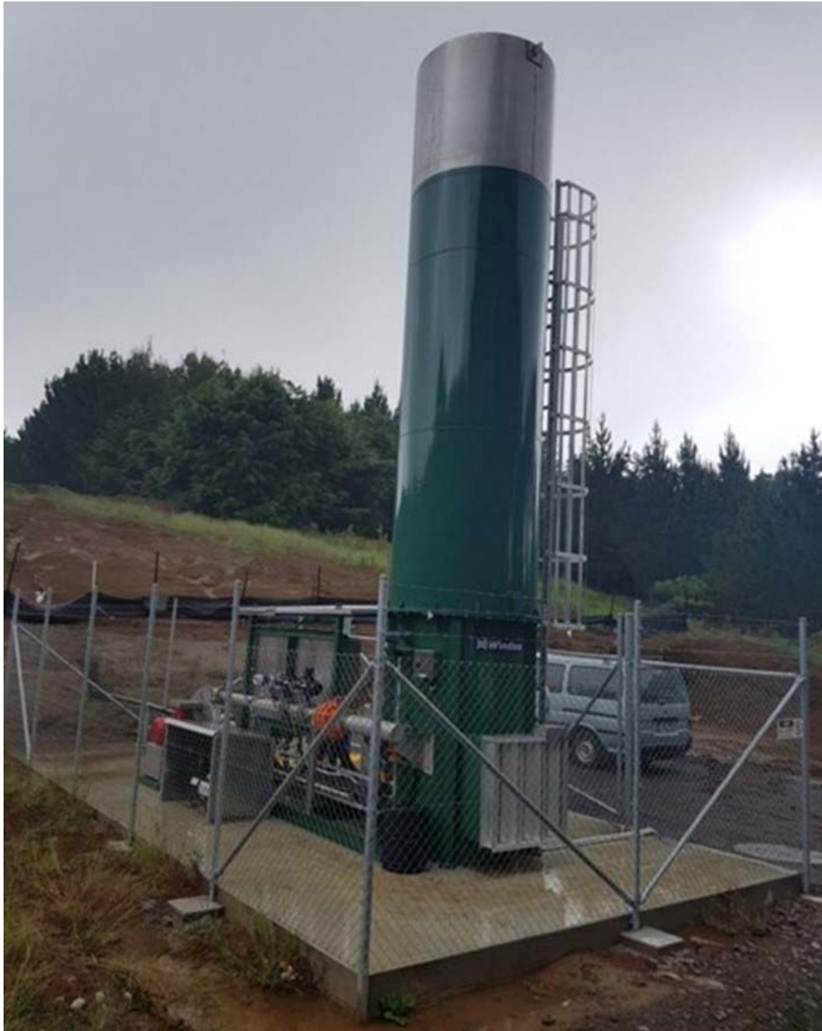
Photo 6 The fully enclosed flare
