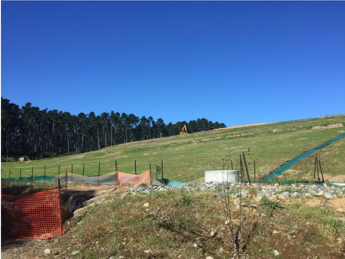
Photo 1 Finished and partially stabilised cap on the northern batter of Stage 3, April 2021
