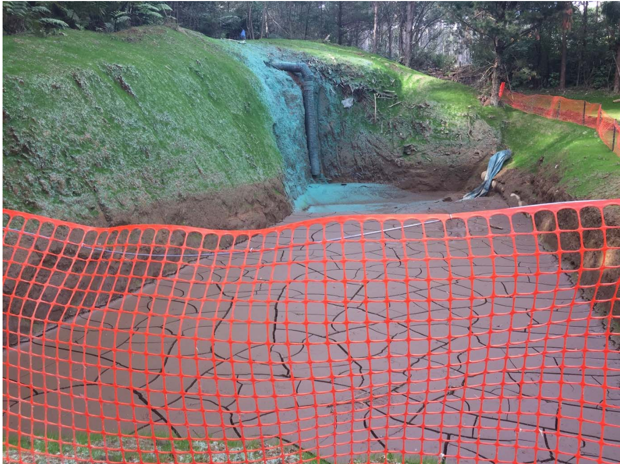
Photo 3 Pretreatment pond for large silt pond, May 2021
