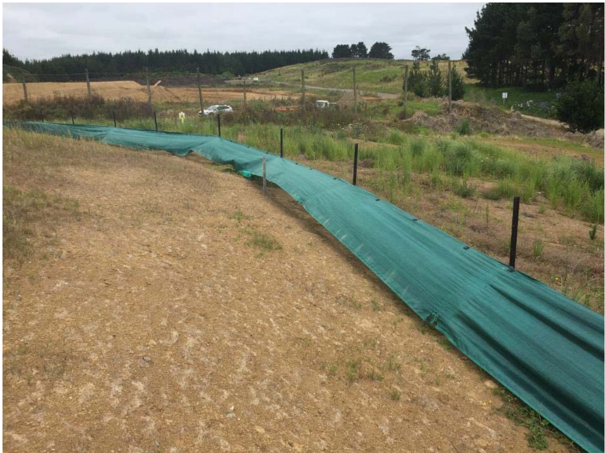
Photo 9 Example of incorrectly installed silt fence 27 January 2021
