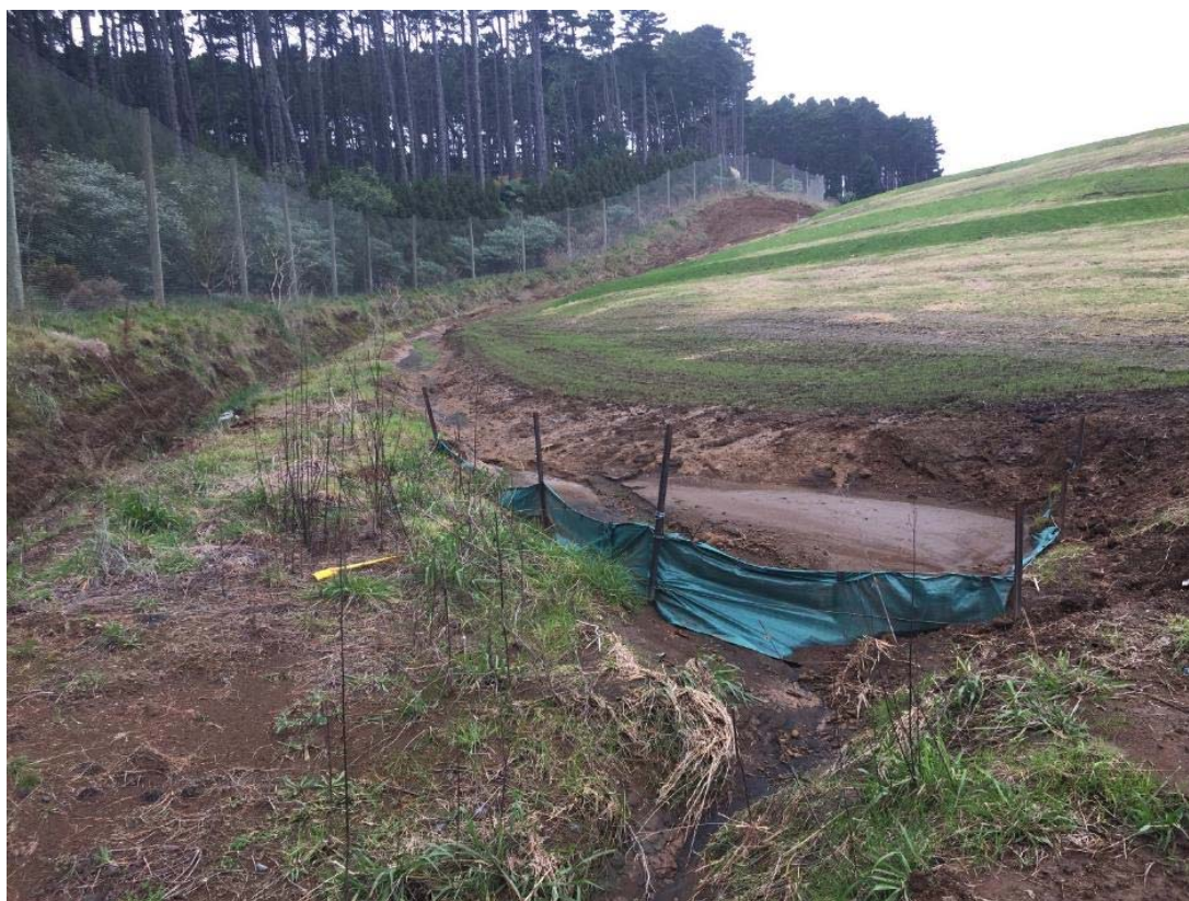
Photo 17 Silt fence requiring maintenance, June 2021
