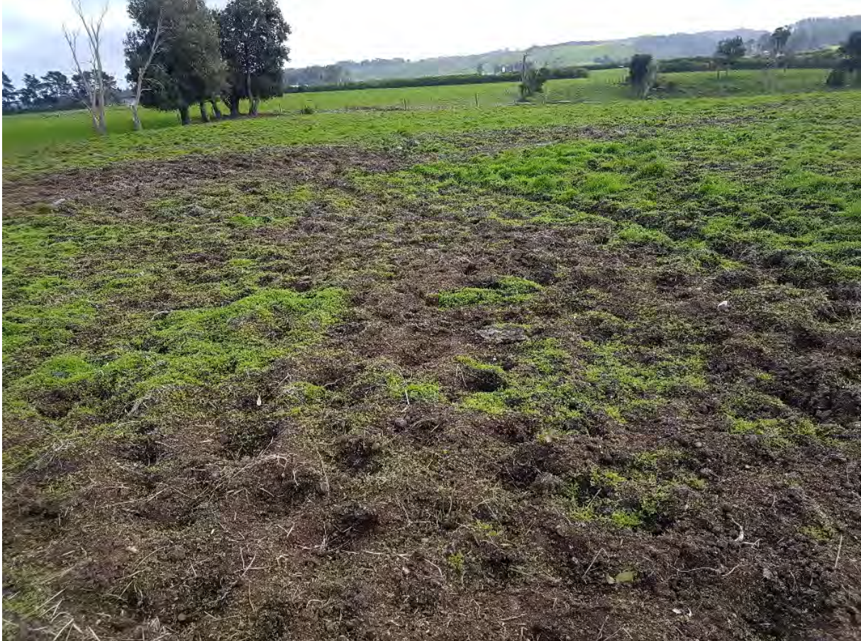
Photo 4 Pugging on filled area that does not have an acceptable final cap, 26 September 2018
