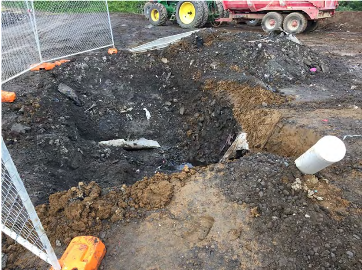
Photo 8 Broken leachate pipe, July 2018
