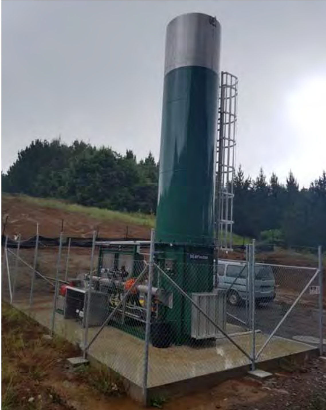
Photo 3 The fully enclosed flare
