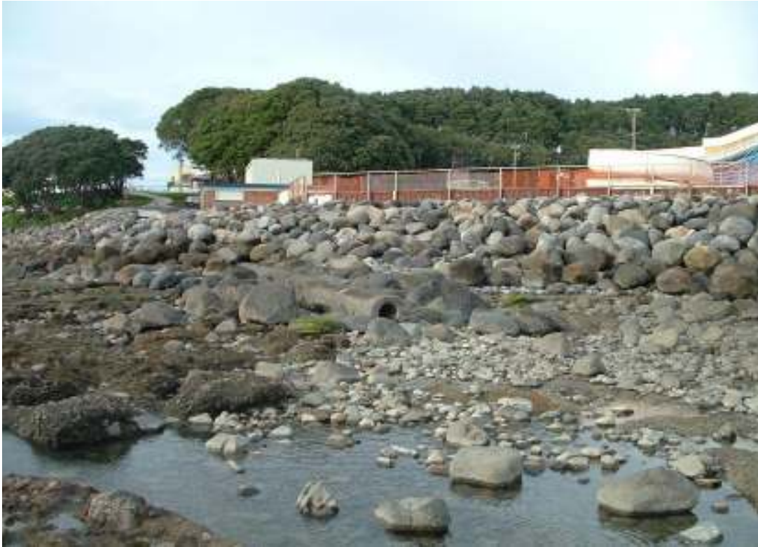
Photo 1 Aquatic Centre marine outfall
