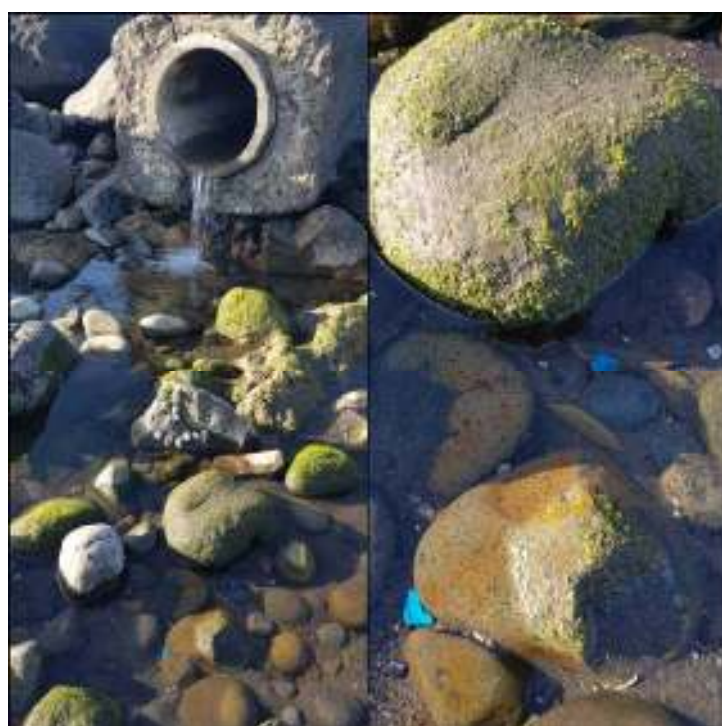
Photo 2 (A) Low flow discharging from outfall at 08:40 (8 May 2018), with blue paint chips visible in the immediate vicinity; (B) Close-up of paint chips
