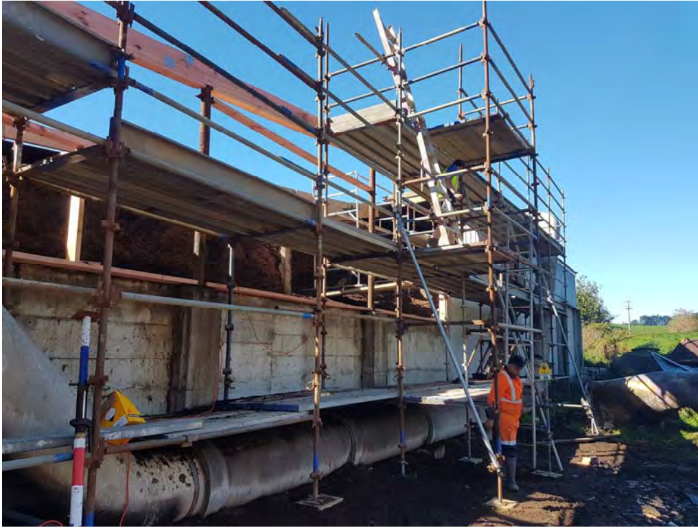
Photo 1 Osflo construction of new rear wall 1 May 2018
