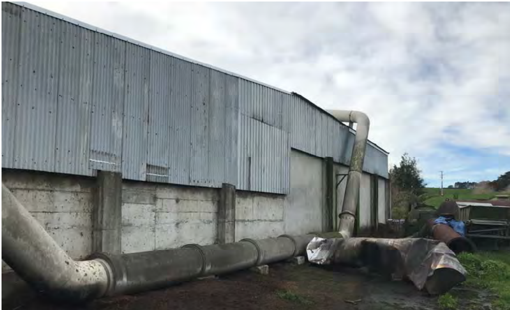
Photo 2 Osflo roof and bio-filter observed 21 June 2018
