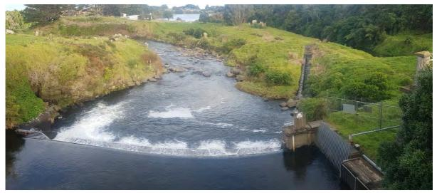
Photo 1 The Waiaua River, weir, intake, canal, fish pass and Lake Opunake, as viewed from the State Highway 45 Bridge, Opunake
