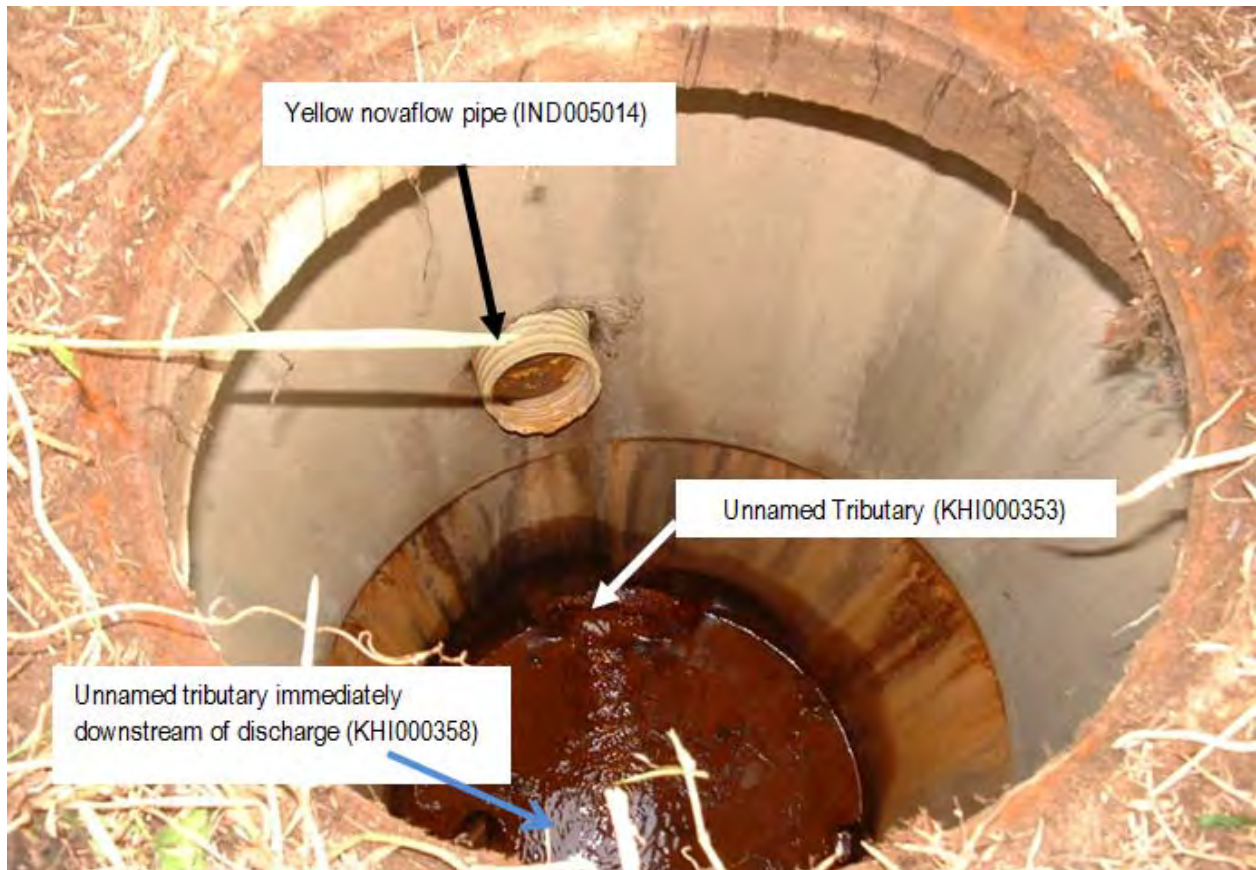
Photo 1 The view down manhole 1 1
