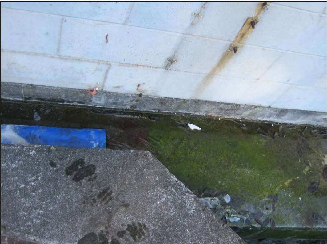
Photo 2 Oil cooling water sampling point
