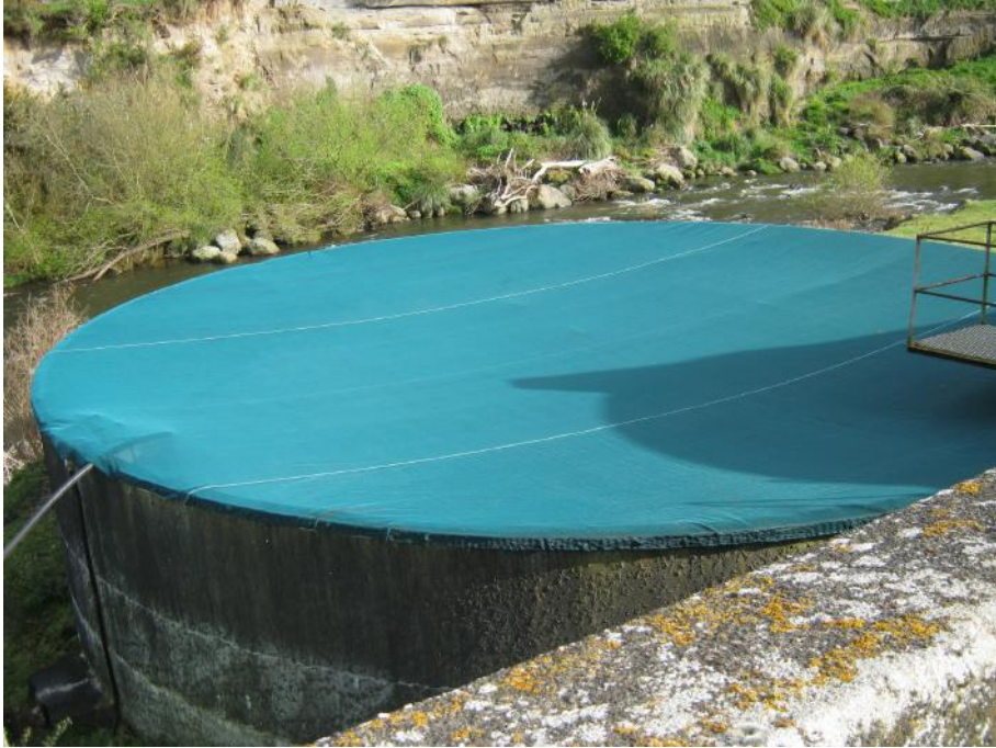
Photograph 1 New cover on the effluent holding tank
