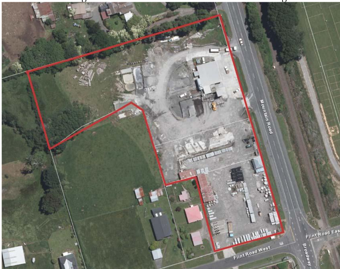
Photo 3 Fletcher Concrete site (Firth Industries and Humes Pipeline systems), Stratford
