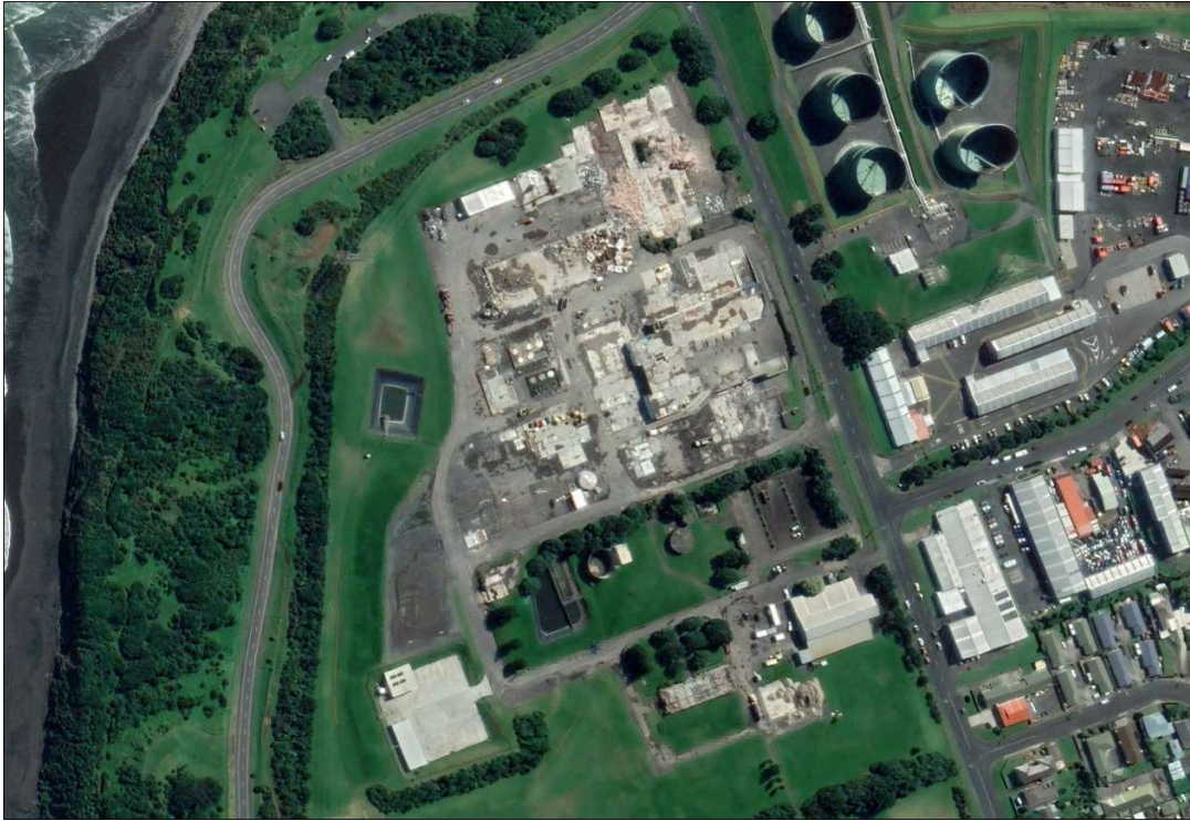
Figure 2: Aerial photograph of the Paritūtū site during demolition, around October 2022.
