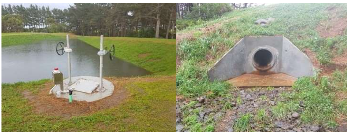
Photo 4 Northern stormwater pond, stop valves and outfall to the Kaupokonui Stream
