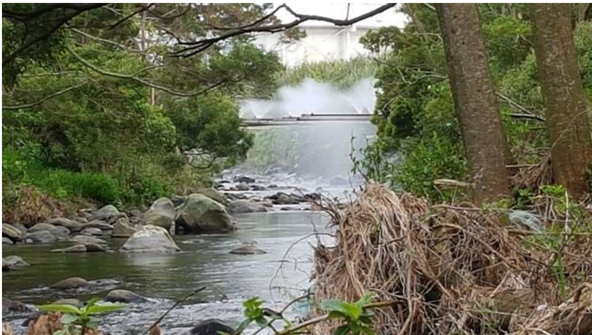
Photo 3 Cooling water spray discharge booms looking upstream from below the discharge area
