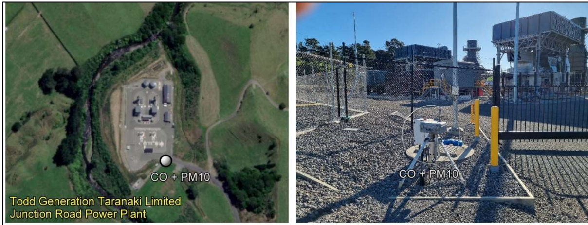
Figure 5 CO, LEL and particulate monitoring site at JRPP (2024)
