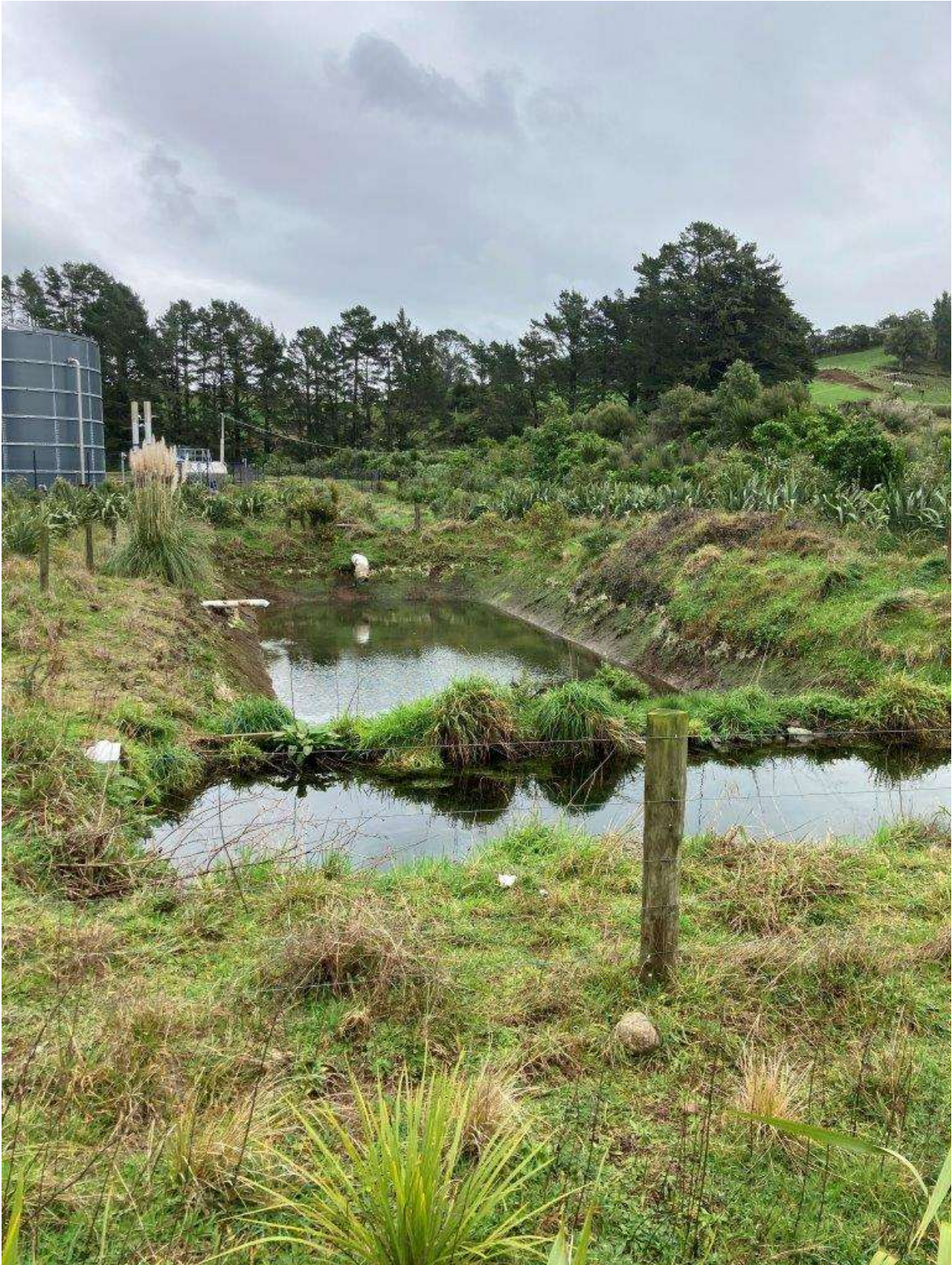
Photo 1 Stormwater sediment/retention ponds system
