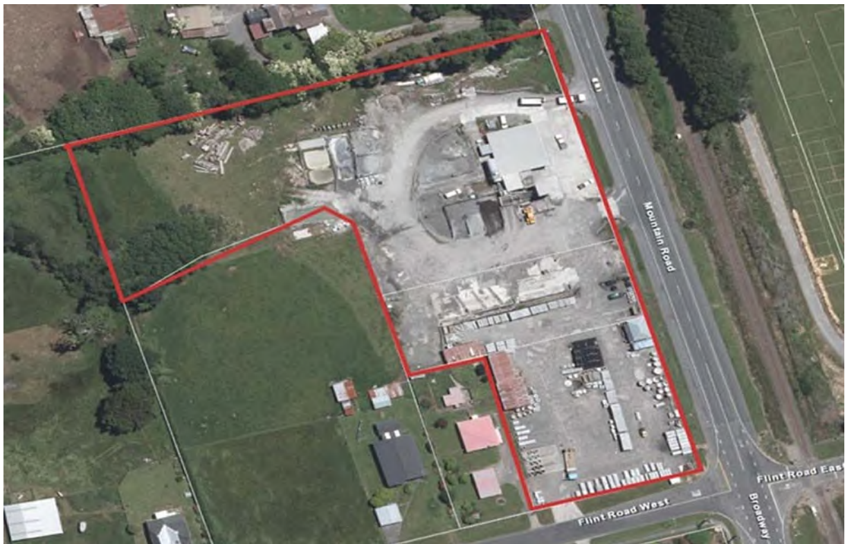
Figure 3 Location of the Fletcher Concrete Firth Industries site, Stratford
