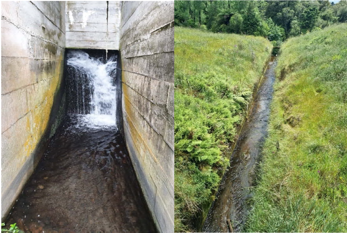
Photo 2 Old sluice gate leak (left (2019-2020)) and race (right (2022-2023))
