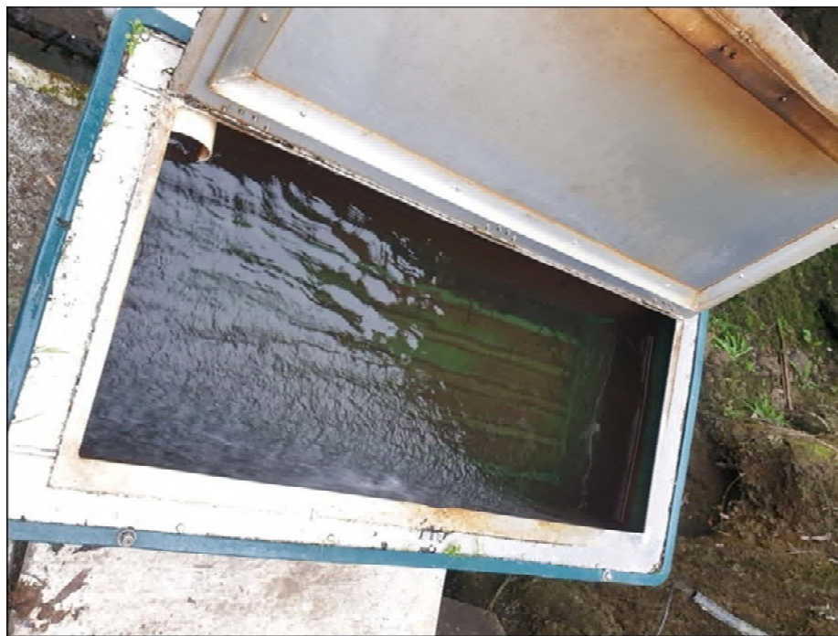
Photo 5 Photo taken of elver in the trap December 2019. Elver enter a pipe carrying the attractant flow, which leads to the trap. These elver are then transferred to an area above the Manganui River head works
