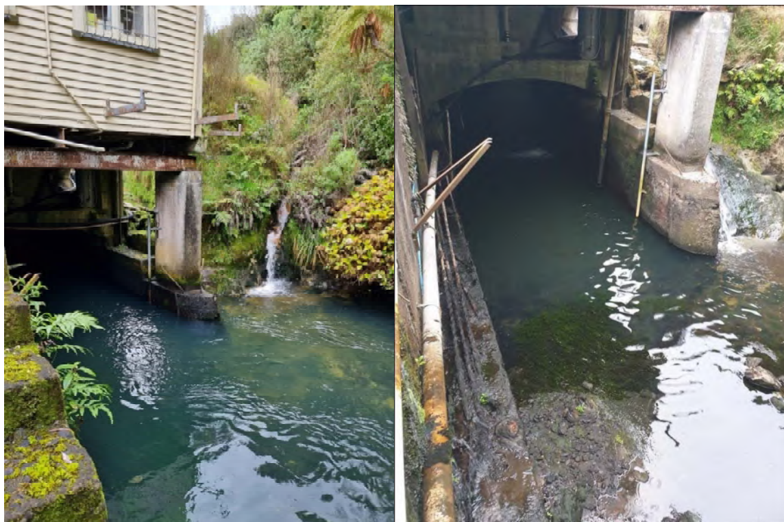
Photo 6 Left photo - Two attractant flows that direct fish away from the trap. One small tributary (right) and one coming from the station (left beside the concrete pillar) (2022-2023). Right photo - there is a third residual flow from the station outlet pipe directly below the building (2019-2020)
