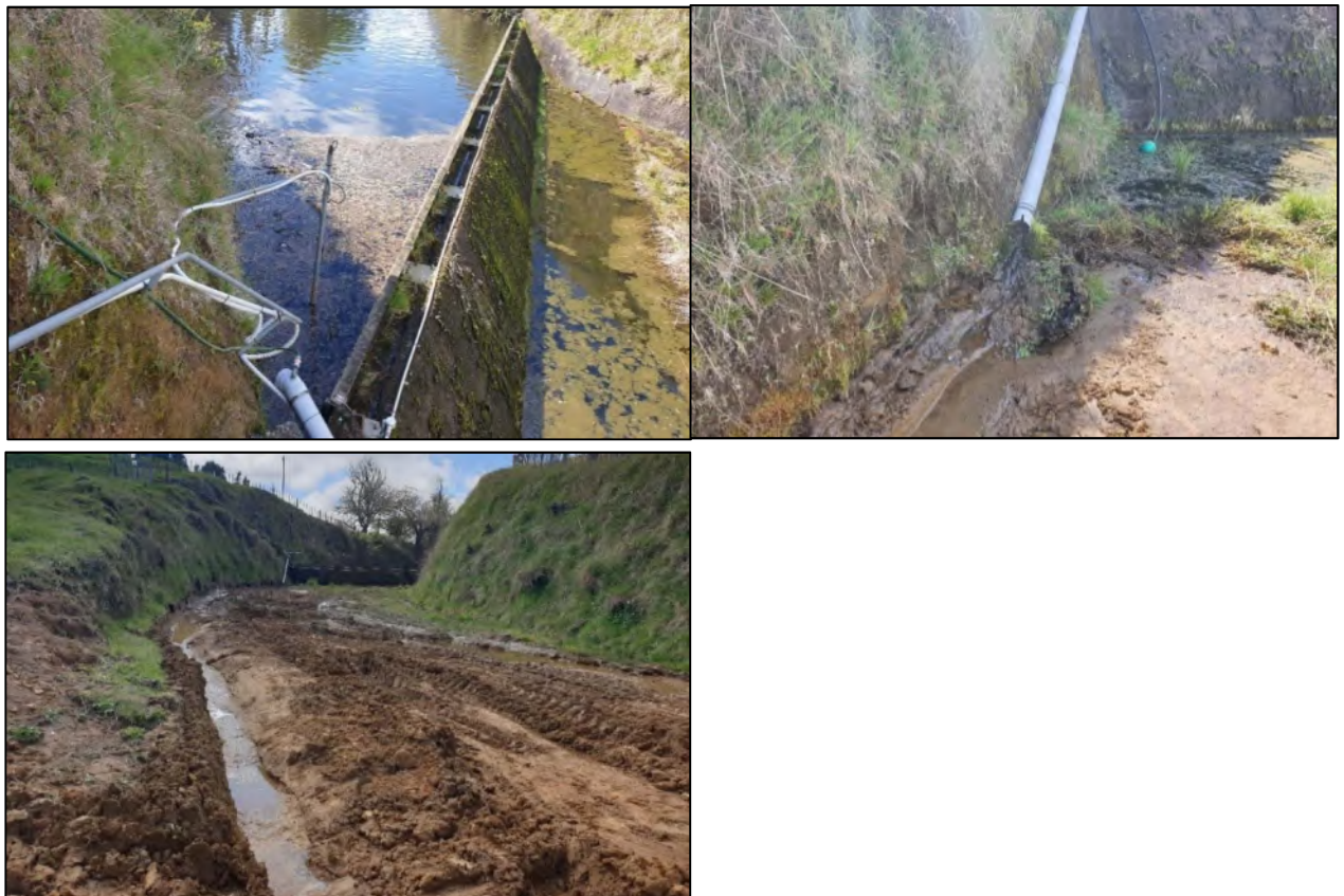
Photo 4 Fish pass at spillway (top left). Fish pass inlet (top right). Fish pass approach through spillway (bottom left). Photos in 2020-2021 compliance period
