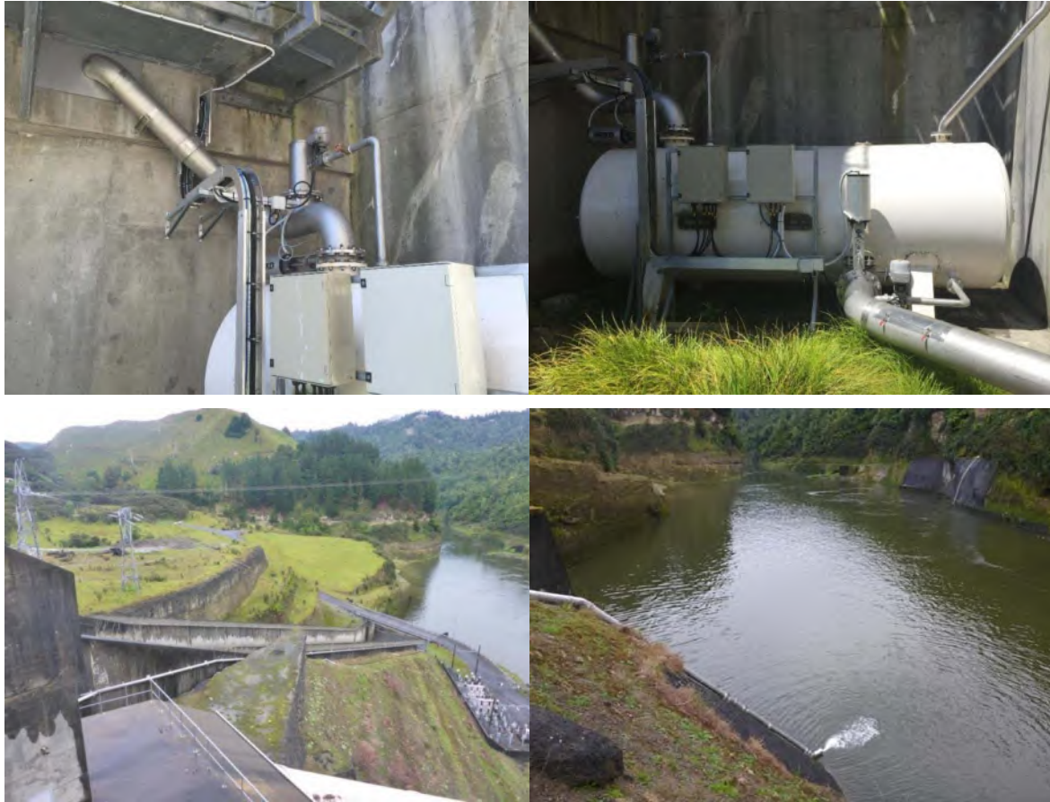
Figure 7 Pātea HEPS eel bypass system
