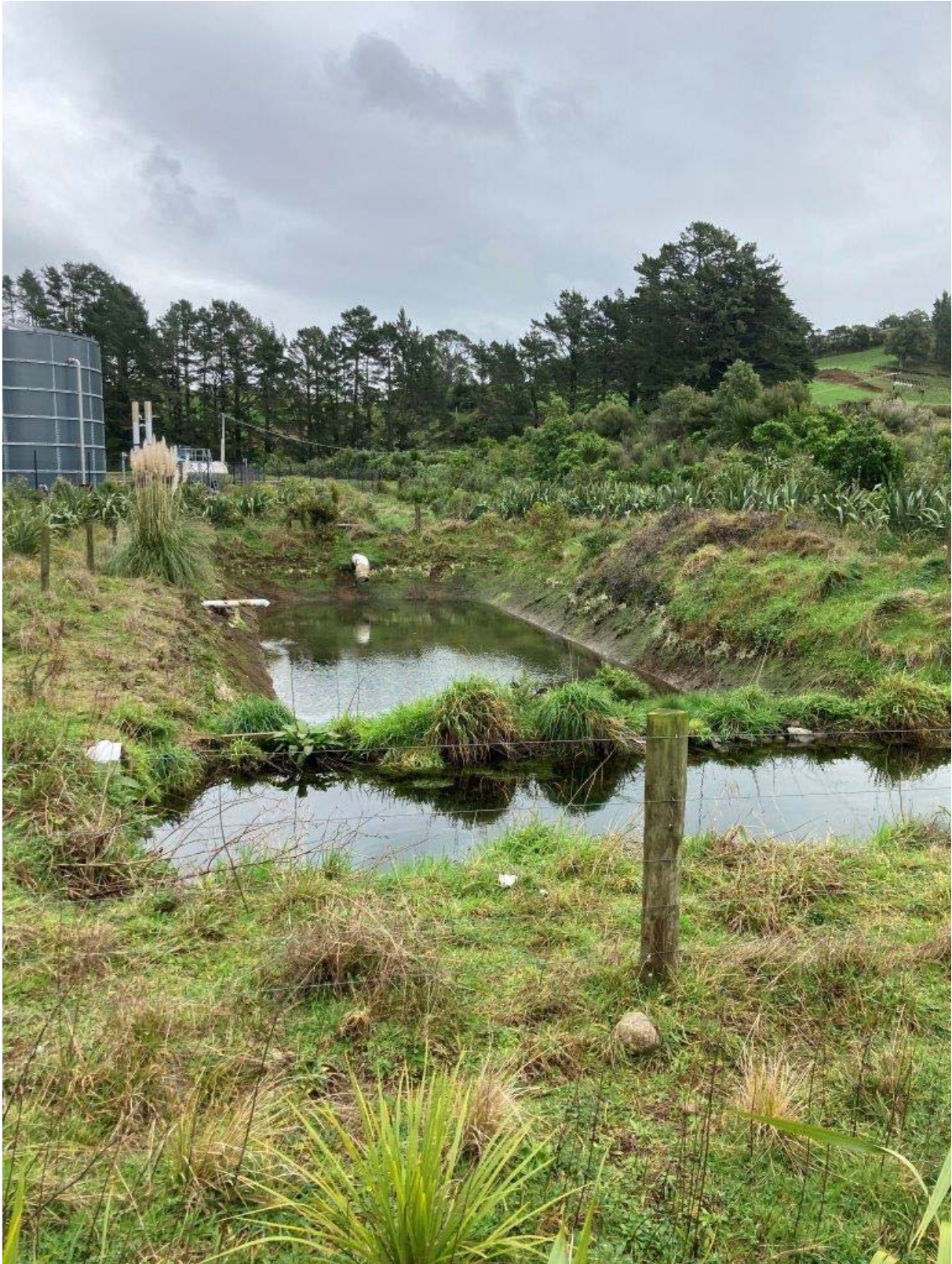
Photo 1 Stormwater sediment/retention ponds system
