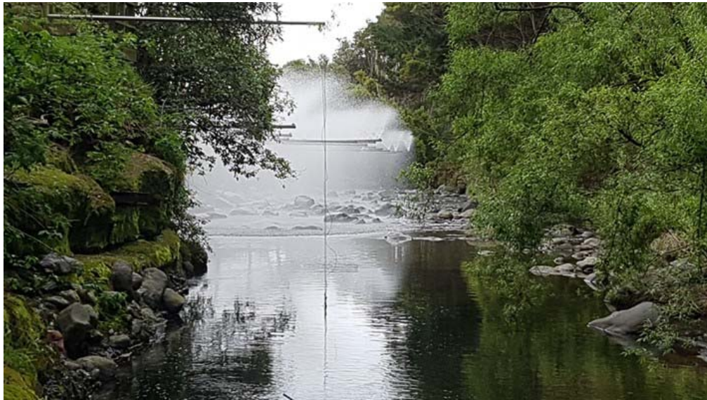
Photo 1 Upstream temperature probe (to May 2023) and cooling water discharge spray booms
