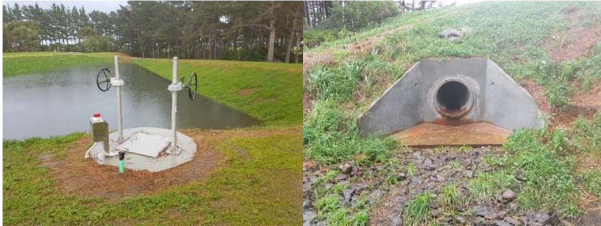
Photo 5 Northern stormwater pond, stop valves and outfall to the Kaipokonui Stream
