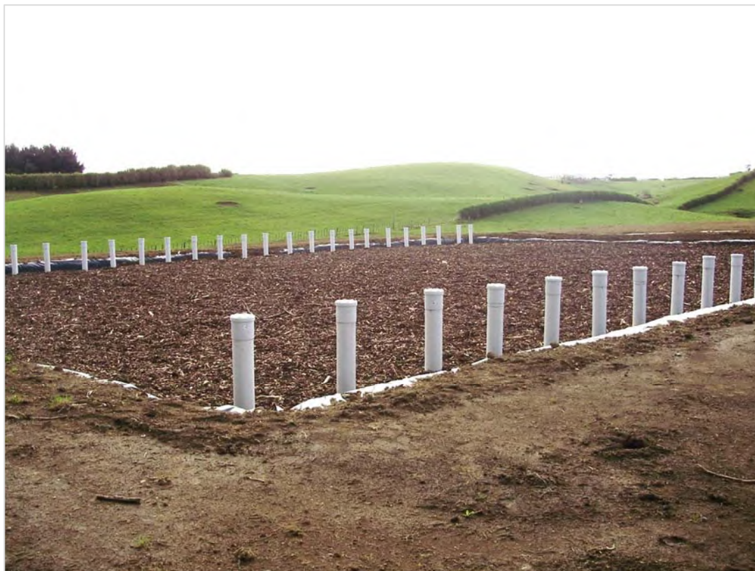
Photo 1 The bio-filter at Graeme Lowe Protein
