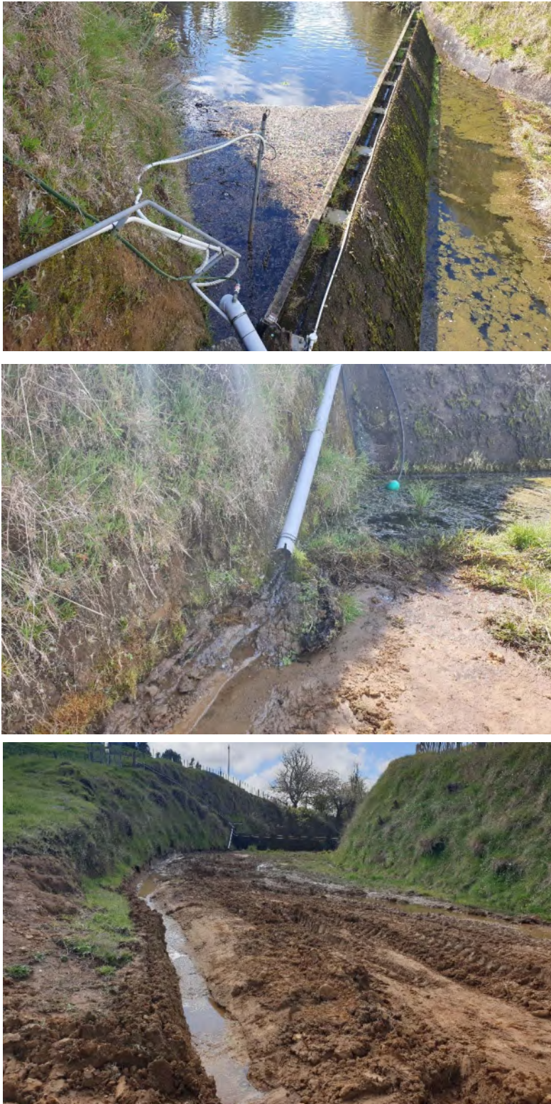
Photo 4 Fish pass at spillway (top). Fish pass inlet (middle). Fish pass approach through spillway (bottom)
