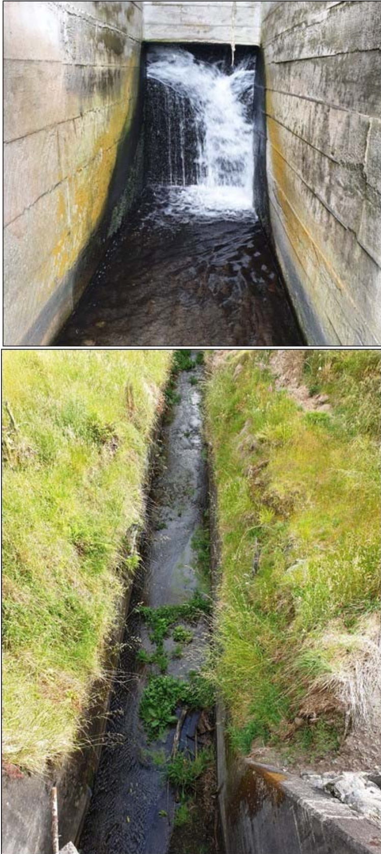
Photo 2 Old sluice gate leak (top) and race (bottom). Photos in 2019-2020 compliance period
